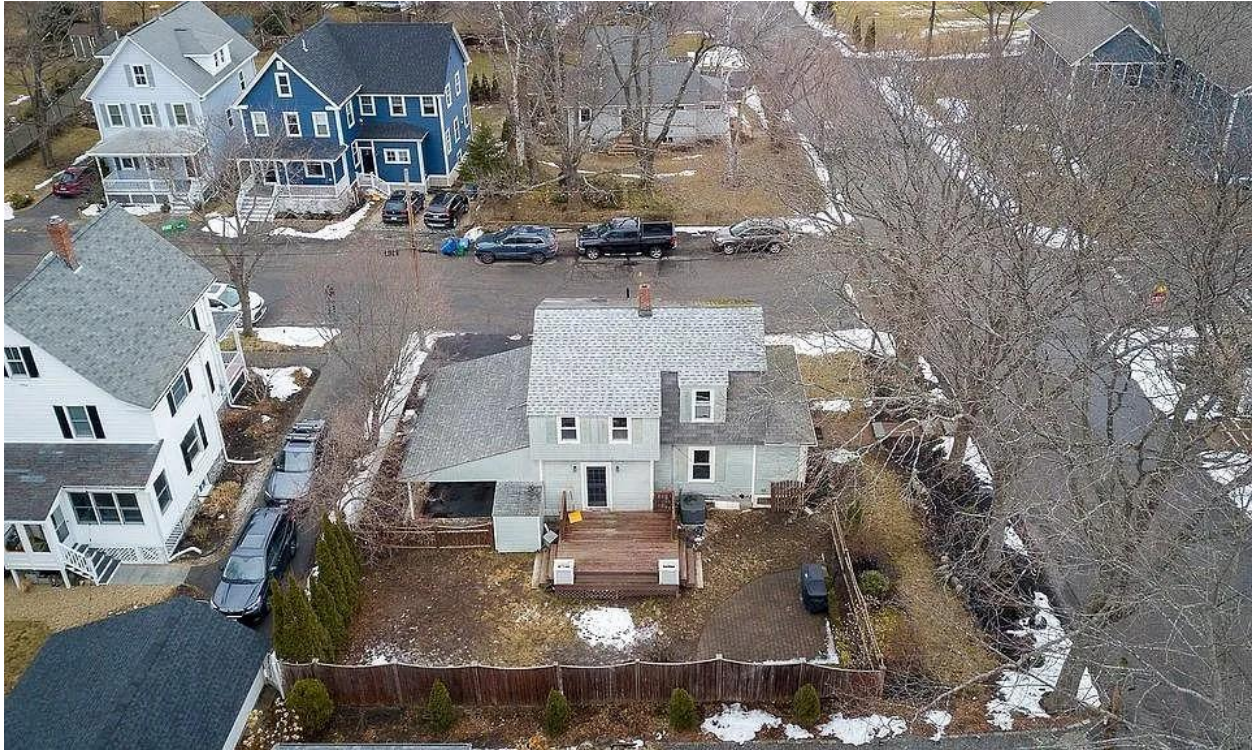
Overhead View (Rear Elevation)
