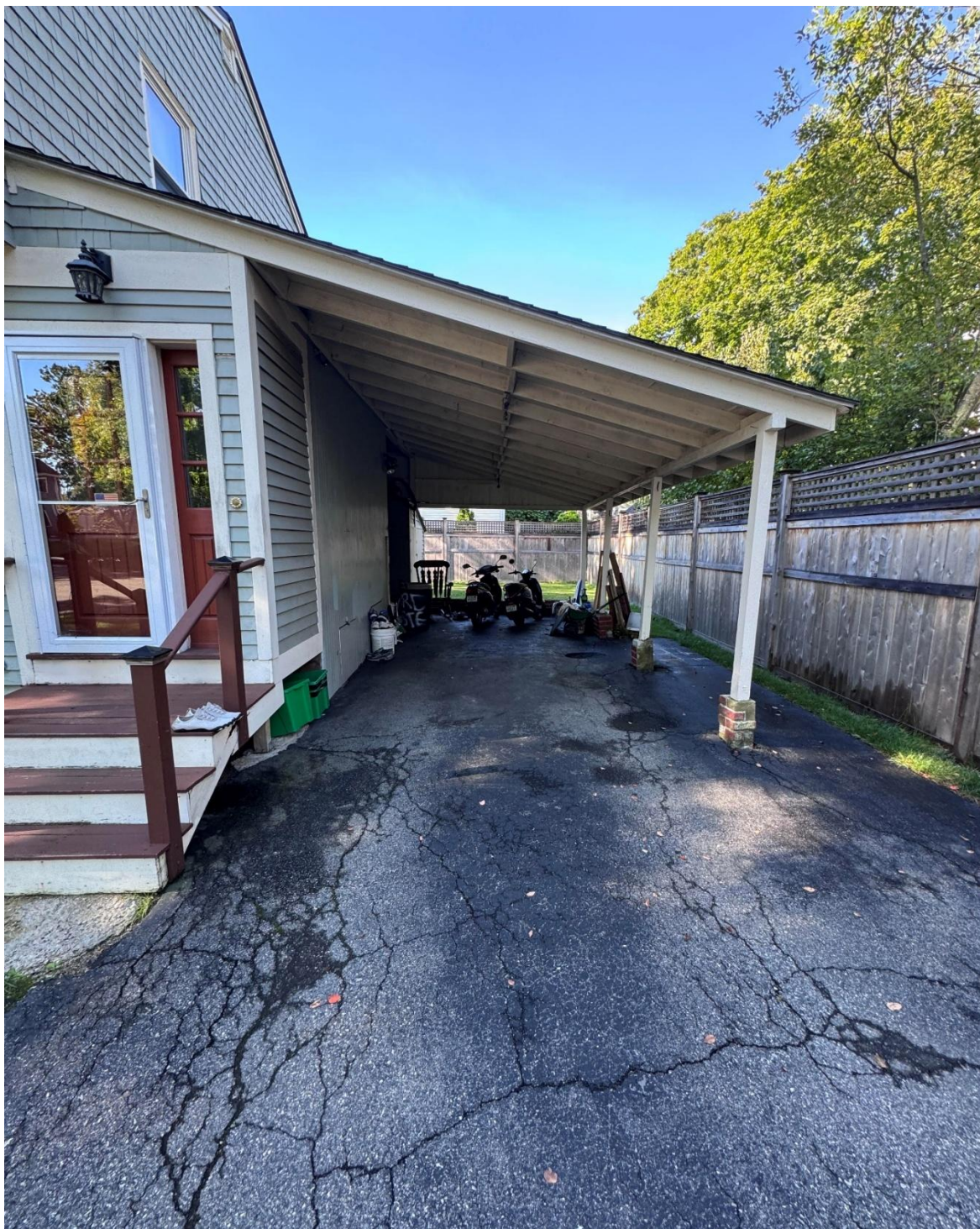
Carport (Sparhawk Street)
