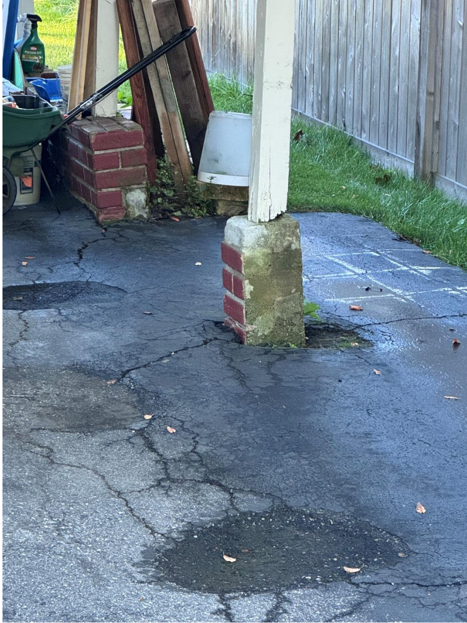
Carport “Structural” Supports
