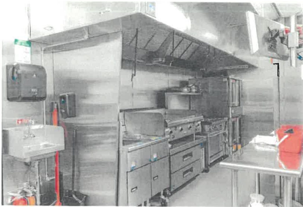
Figure 15: Additional kitchen detail
