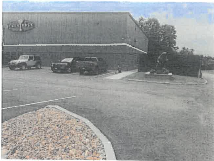
Figure 3: Front and right side of building, looking west.
