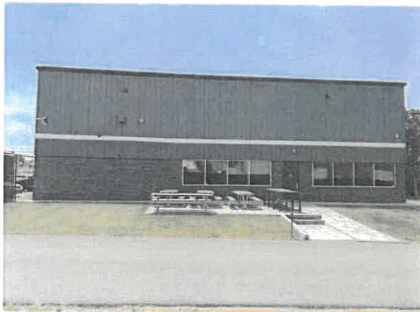
Figure 4: Right side of building, looking south.
