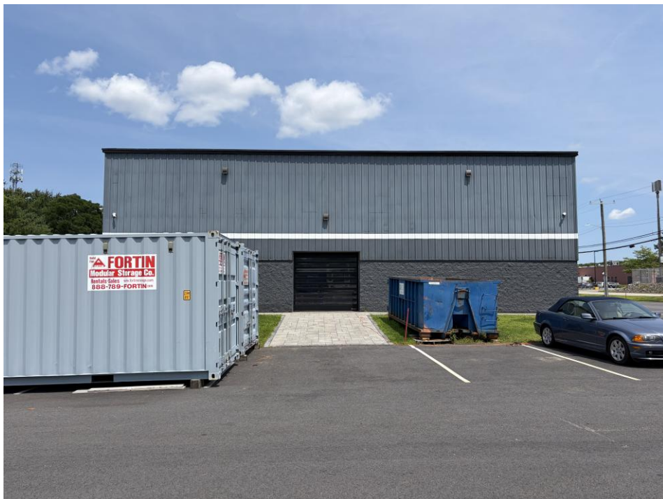
Figure 6: Left side of building, looking north.
