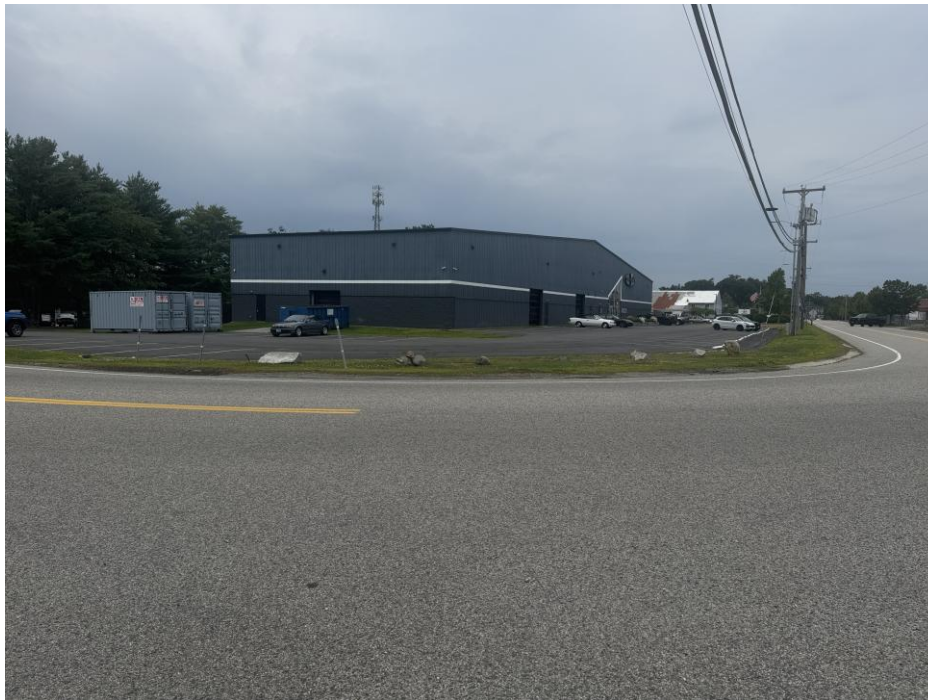
Figure 2: Front and left side of building, on West Road looking northwest.
