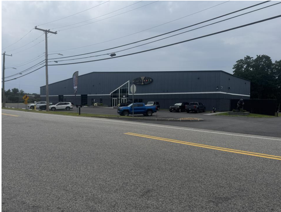
Figure 1: Front of building, on West Road looking southwest.
