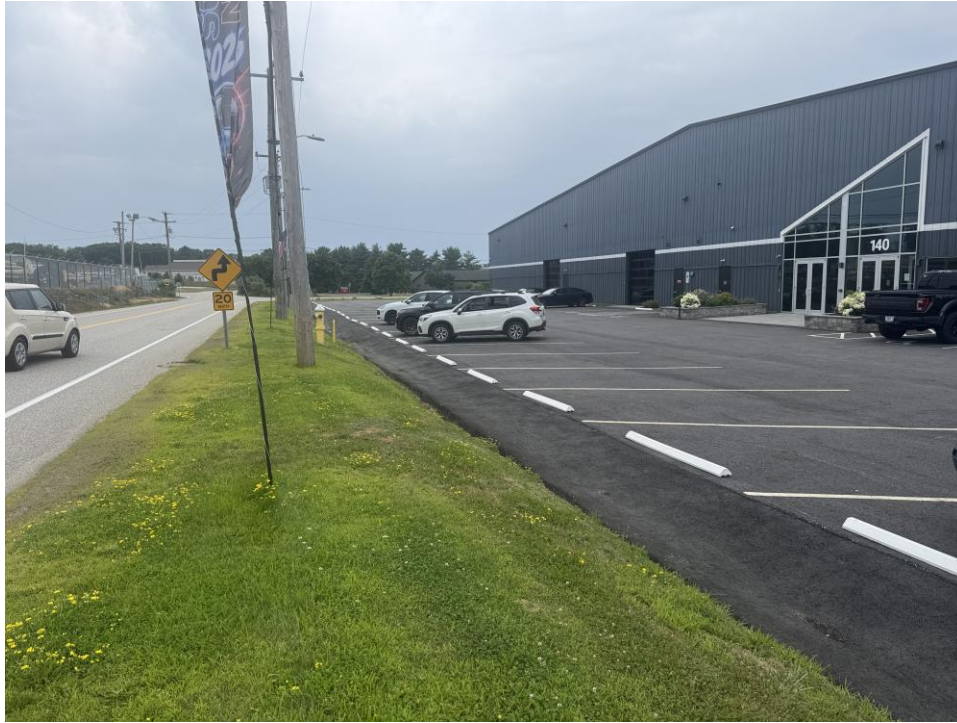
Figure 7: Front parking lot, looking south.
