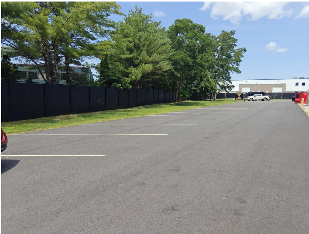
Figure 10: Rear parking lot, looking northwest.
