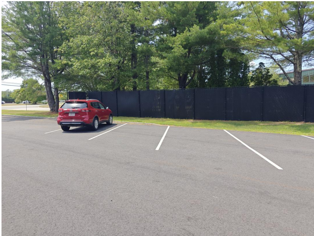
Figure 12: Fence on rear of site, looking west.
