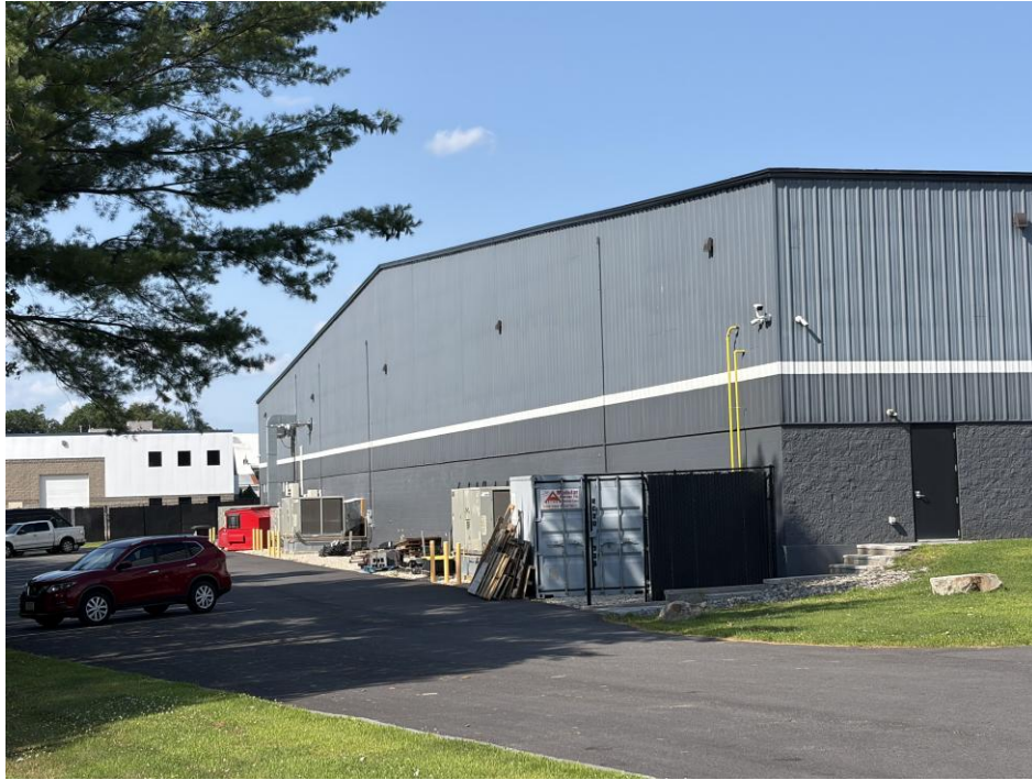
Figure 5: Rear of building, on West Road looking northeast.
