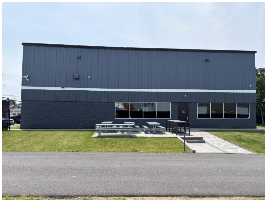
Figure 4: Right side of building, looking south.
