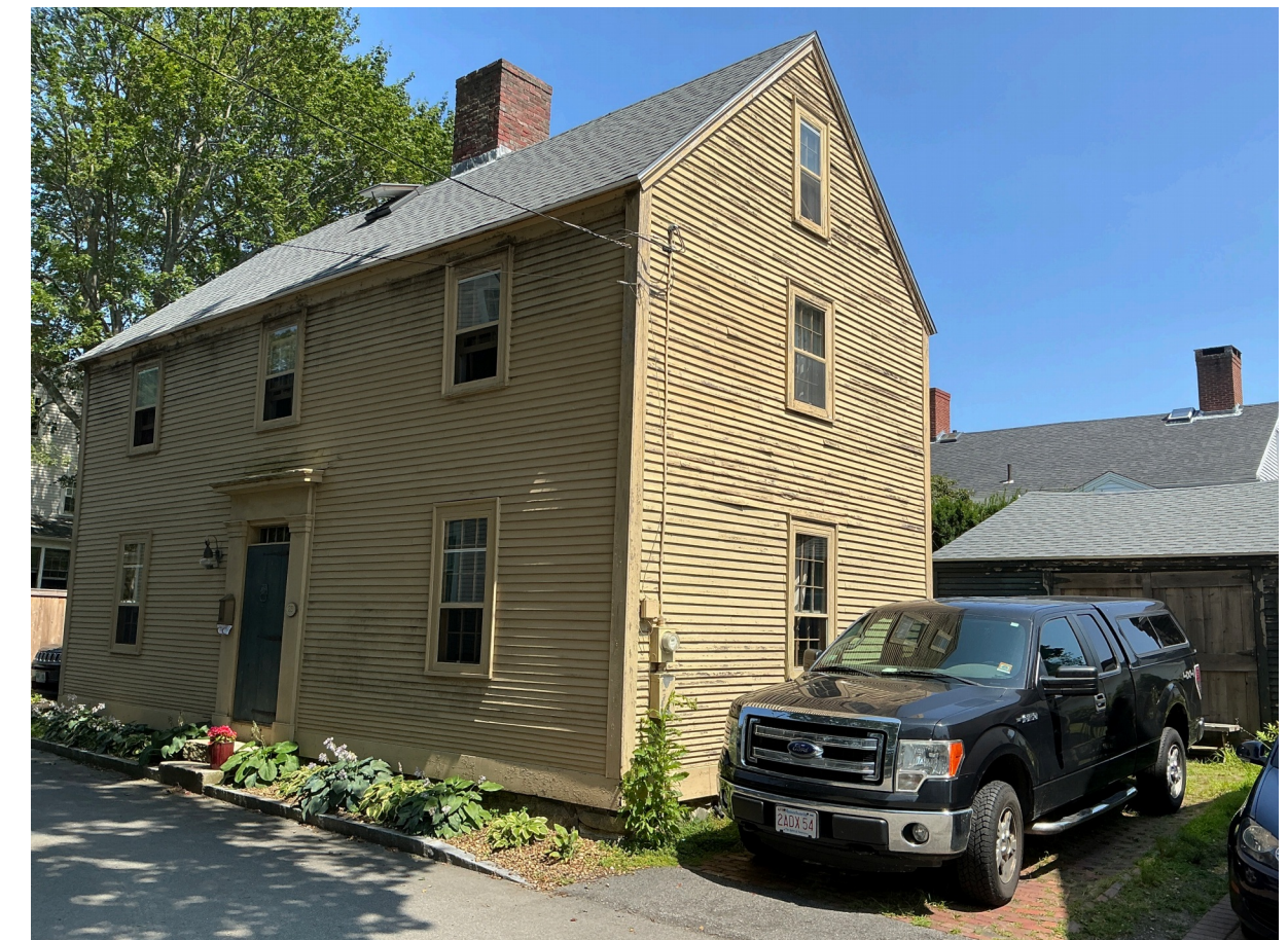
EXISTING FRONT VIEW
