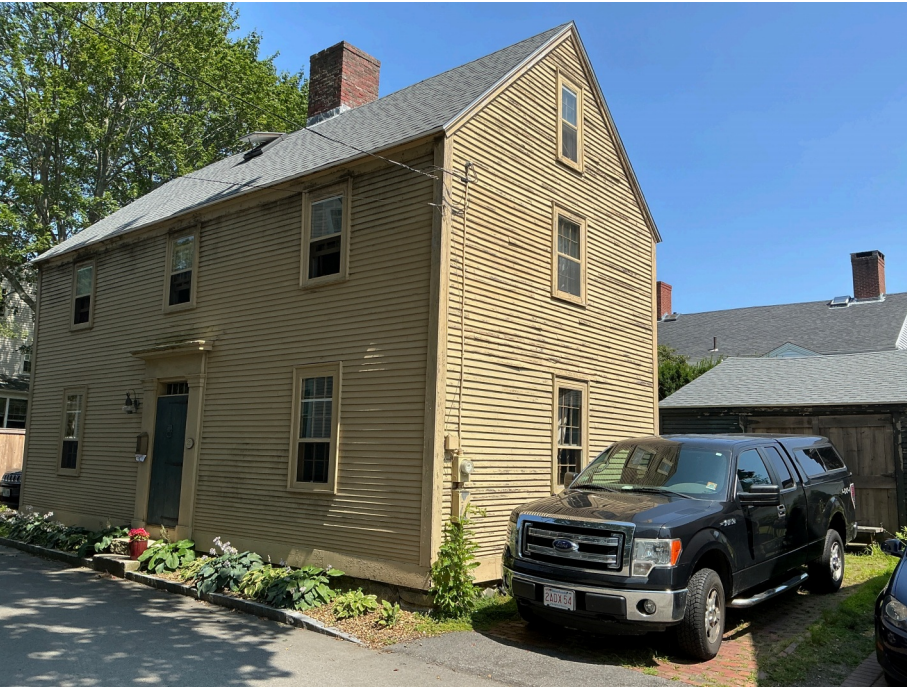
EXISTING CONDITION PHOTO
