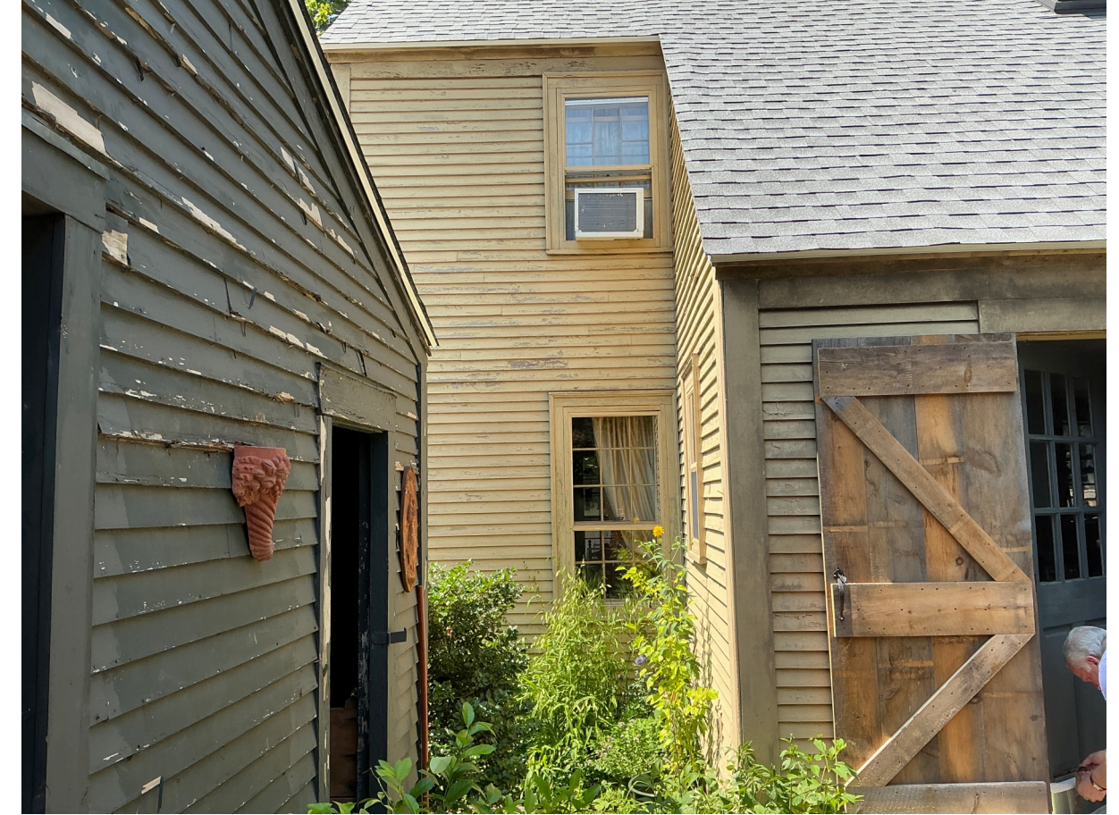
EXISTING REAR VIEW
