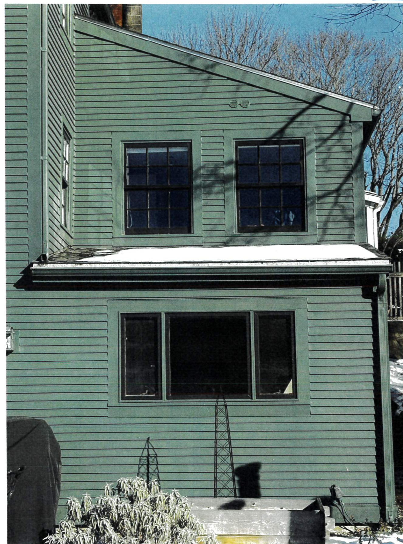
South Elevation: close-up of existing one-story addition
