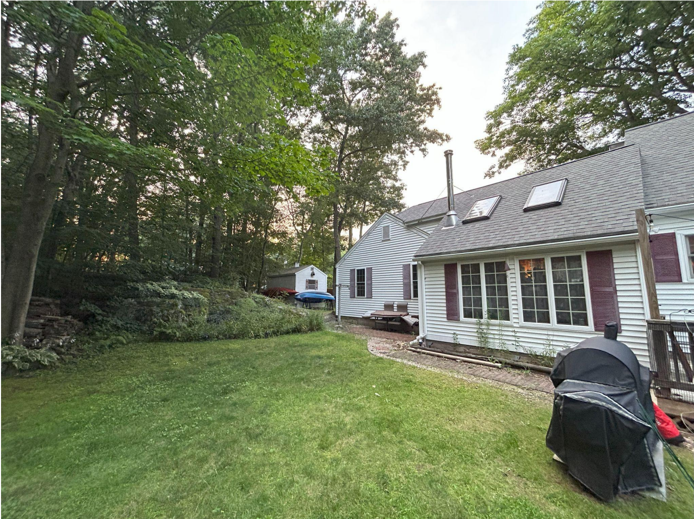
Property Photo #4 - View of Breezeway wall looking NW.
