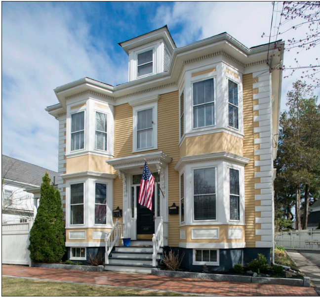
Identification of key building features, such as the symmetrical façade, two-story projecting bays and projecting cornice can help identify where and to what extent alterations may be appropriate.
