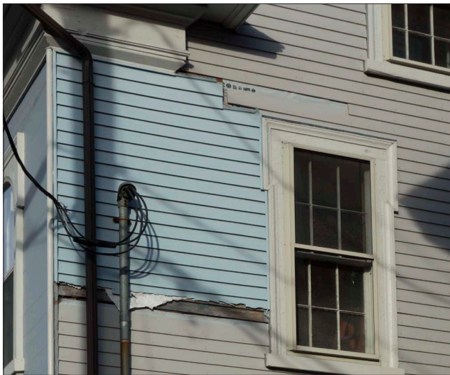
The removal of vinyl or aluminum siding can reveal underlying wood siding, shingles and trim.
