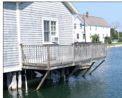
Unlike porches, which were designed as an integral component of a building, decks are generally made from stock lumber and are not stylistically integrated with historic buildings. As a result, their visibility should be limited from the public right-of-way.
