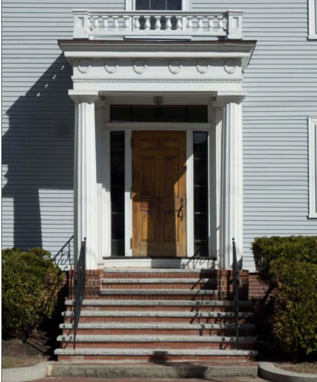
An entrance porch can evoke a sense of grandeur and provide a welcoming feature for visitors.
