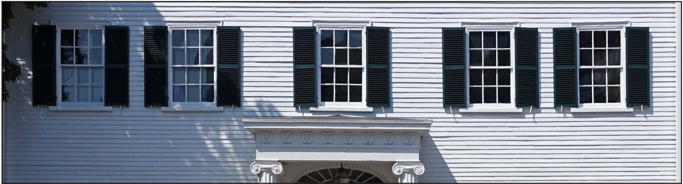
Center-hall homes generally have a single window centered over the door flanked by a pair of windows at each level. In this example, the windows all have 6/6 double-hung sash with wood louvered shutters.
