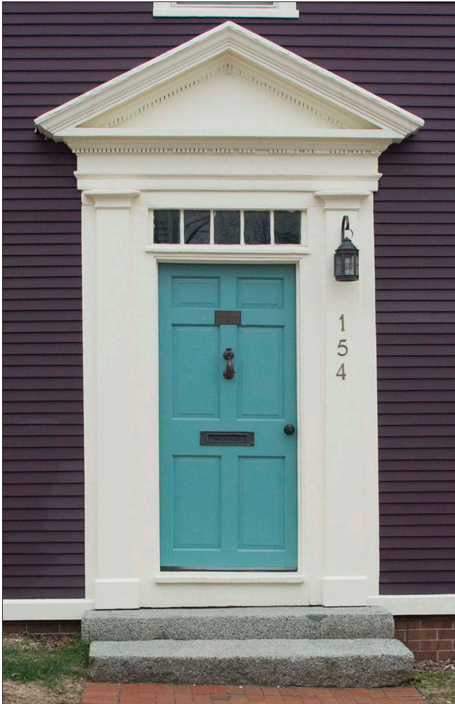
Most of the doors found at historic homes in Portsmouth are paneled wood. This example includes a multi-light transom window and pedimented door surround.
