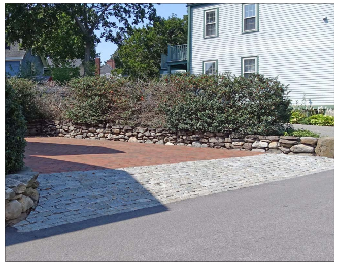
The parking area is brick and the driveway apron is made from cobblestones. The parking area is flanked by dry-laid stone walls, and shrubs provide a visual separation with the neighboring property.
