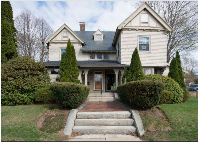
Steps in the landscape provide pedestrian access where there are changes in grade on a site. This example includes granite steps and curbing flanking a brick walkway.
