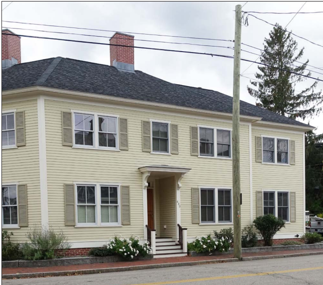
The massing and materials at this new building are similar to historic buildings in the area, however the design would be more sympathetic if the shutters were sized to fit the window openings and if the windows were separated.
