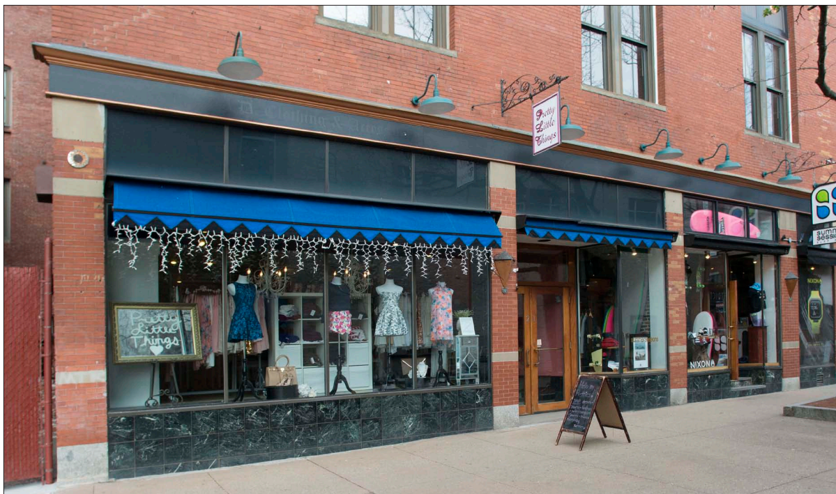
The storefront of these shops is visually separated from the upper portion of the building by a storefront cornice. Projecting signs for each of the businesses are suspended from brackets located below the second floor windowsills. A series of gooseneck lights extend above all of the storefronts to provide sidewalk illumination.
