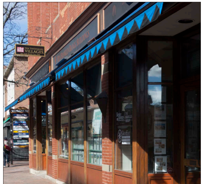
Consistent signs and awnings along this row of shops provides a visual separation between the storefronts and offices above.
