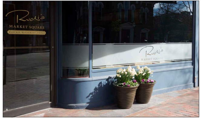
The entrance door includes a gold leaf sign with the restaurant name. The frosted applique shields direct view of diners while the majority of the glass remains clear.
