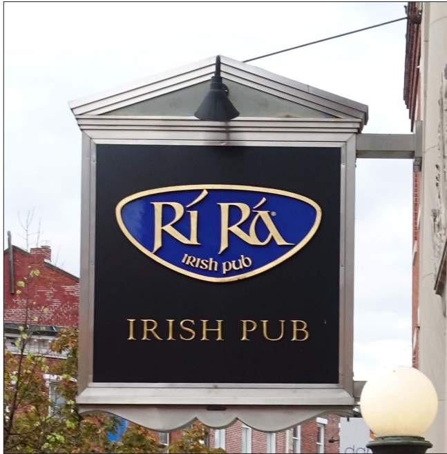
The restaurant reused the frame from the former bank, saving an important architectural feature. Indirect lighting is provided by a gooseneck light at each side.
