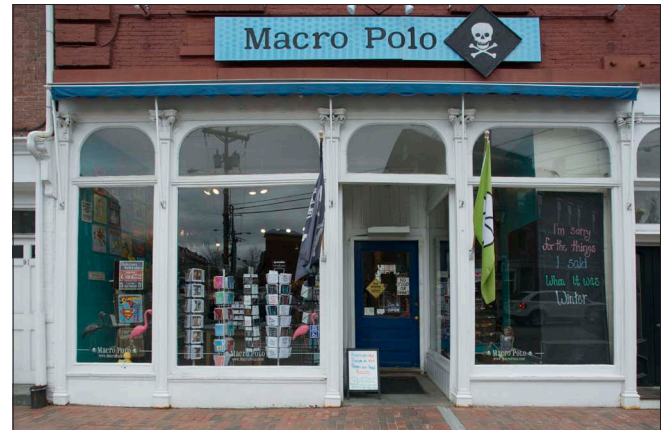
A common feature of many commercial properties in Portsmouth is a storefront. This example include arched transom windows, a recessed entrance alcove, and decorative supports flanking display windows.
