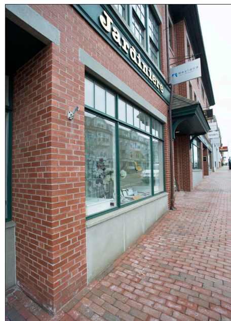
The majority of buildings in the downtown area of the Portsmouth Historic District are masonry, combining brick and stone, and many have highly ornate details, particularly at the cornice. The storefront windows have large, divided lights with exterior muntins, giving them the appearance of wood.
