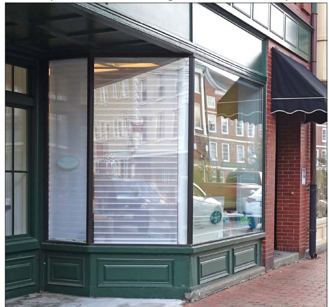
The use of curtains allows the flexibility of privacy for certain areas within the building, while other areas are open to view.
