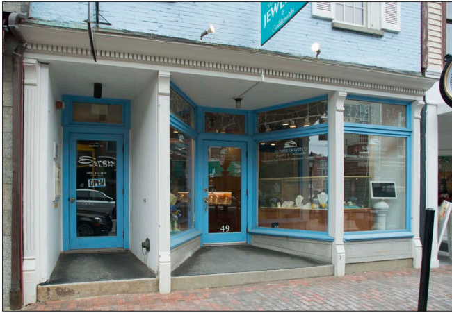
Two entrance alcoves provide access to the ground floor retail and upper building floors. The alcoves provide protection from the elements and increase the retail display frontage. Display windows and doors are topped with transom windows. Fluted structural supports are topped by a decorative storefront cornice.
