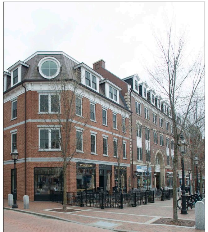
Although this is a large-scale building, it successfully combines elements of traditional architecture with modern elements in a manner that makes it highly consistent with its surroundings. This includes a prominent cornice, punched windows, a brick facade with contrasting cast stone elements and ground floor storefronts along the streetscape.
