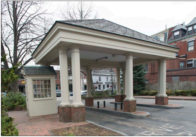
Using traditional materials, trim and details at a non-historic element, such as this bank drive-through and guard booth, can make a modern element more consistent or compatible with the surrounding context.
