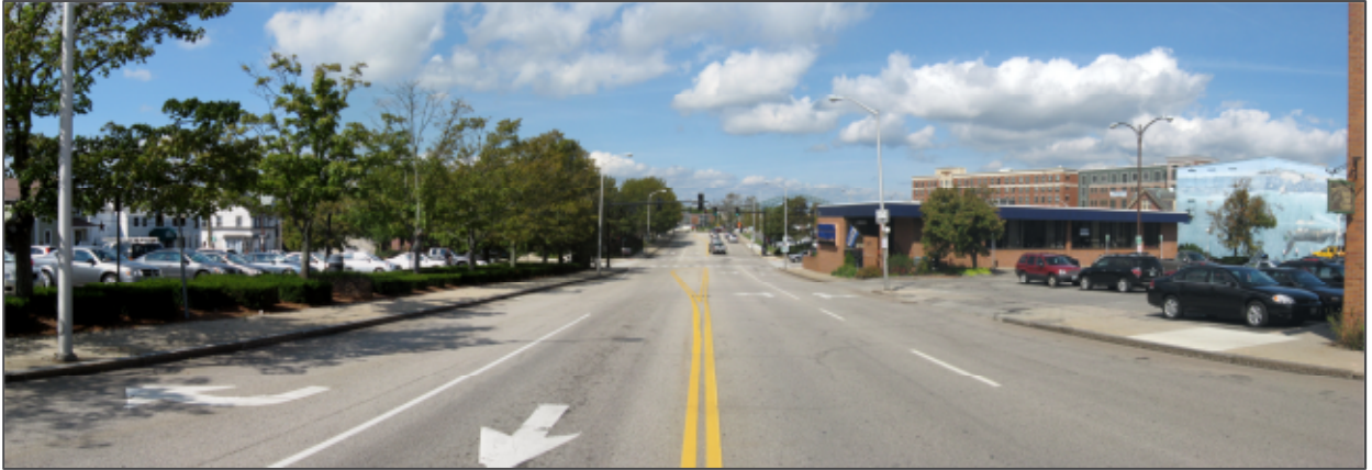
FIGURE 2: MAPLEWOOD AVENUE LOOKING EAST
