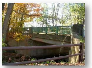
**Description**: This bridge is beyond its 50-year design life. It cannot handle heavy truck volumes and loads. The bridge needs to be replaced. Residents have asked for the bridge to remain open if the median on Route 1 Bypass is extended past Cottage Street. This ensures emergency vehicle access to the Portsmouth Hospital from the neighborhood.
