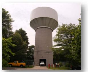
**Description**: The City owns and operates four water storage tanks. These facilities are inspected routinely for the condition of the interior and exterior finishes. Funding covers the costs to repaint the tanks when needed. FY23 funds will be used to repaint the Spinney Road tank.
