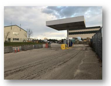
**Description**: Replacement of the fuel station at the DPW including replacement of the underground fuel storage tanks, fuel dispenser island, fuel dispensers, canopy, and telemetry system. Existing fuel tanks have reached the end of their useful lifespan.
