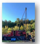
**Description**: This project consists of constructing, permitting and connecting a new groundwater supply well, adjacent to the existing Collins Well, into the Portsmouth water system. This project is important to ensure long-term sustainability of the water supply.
