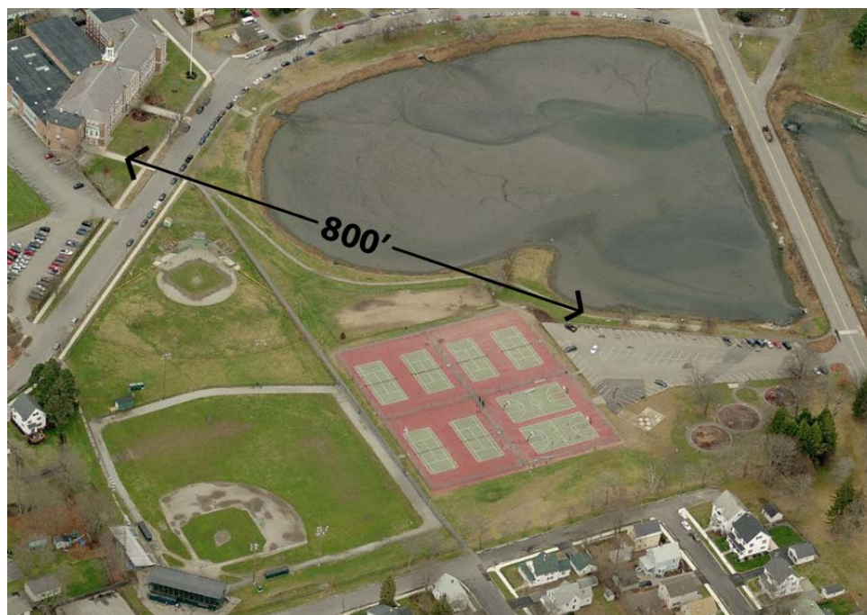
The new drop-off/pick-up zone for parents and students in private automobiles is recommended for City-owned parking lot less than a ¼ mile from the middle school (aerial photo from www.bing.com/maps )
