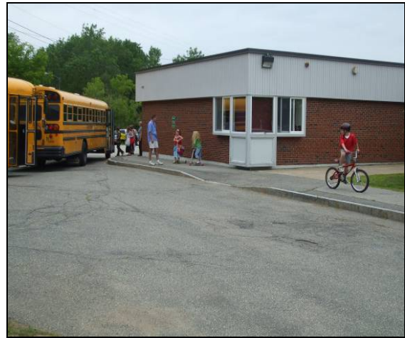
Currently, buses are able to drop students off at the curb very close to the entry of the school
