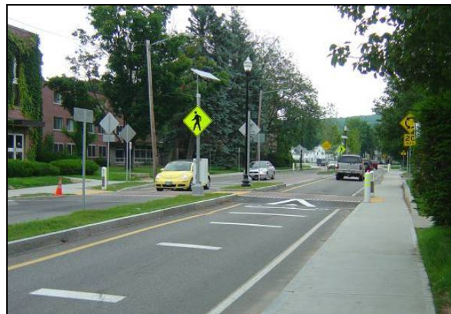
Raised crosswalks, like this one near the Keene State College campus, effectively slow traffic near schools and facilitate safe pedestrian crossing.
