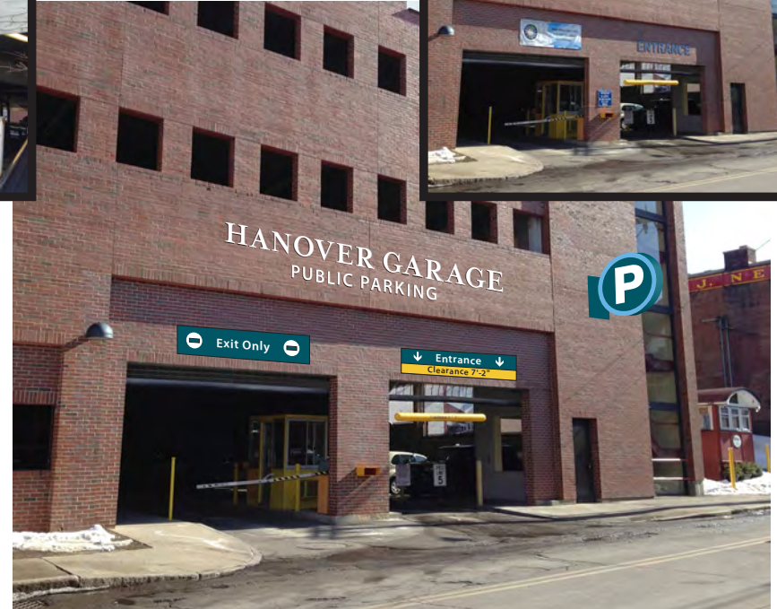
Secondary Hanover Garage Entrance: Fleet Street
