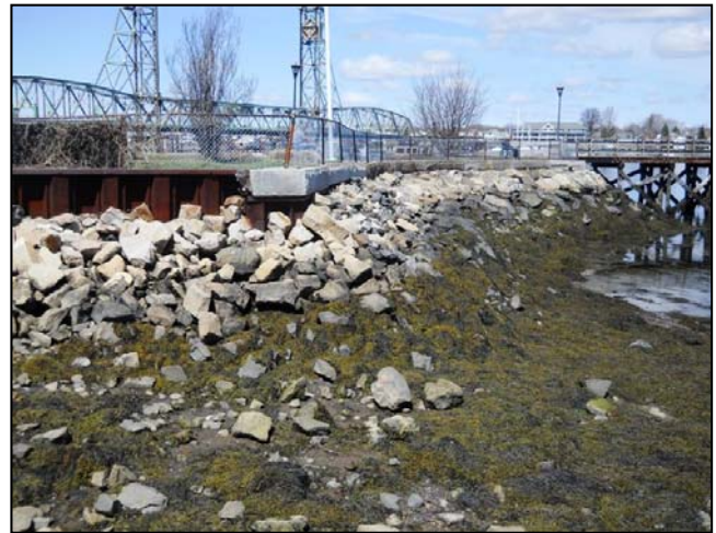
Photo 12: Steel sheet pile bulkhead south of T-Head Pier
