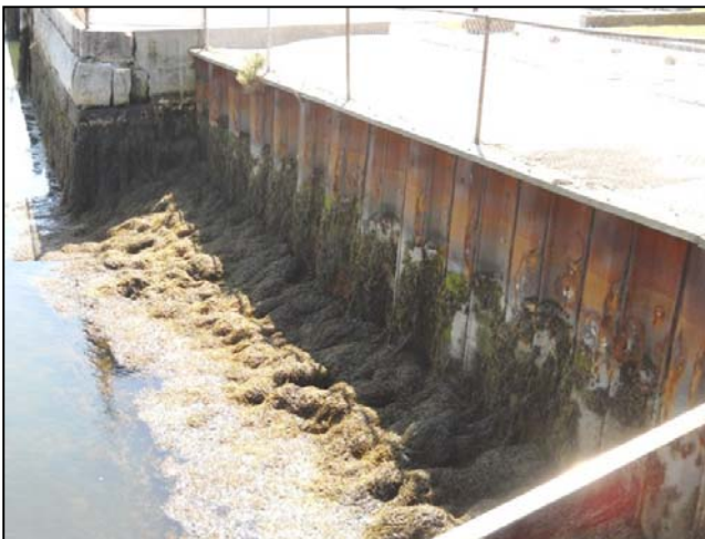
Photo 11: Steel sheet pile bulkhead at North Pier
