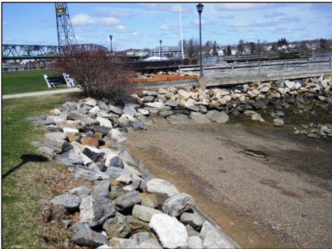
Photo 13: Riprap slope at South Pier
