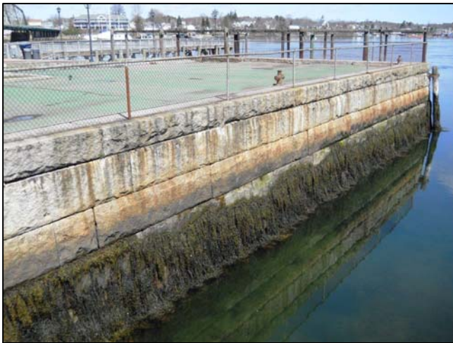
Photo 9: Quaywall at Basin Looking North
