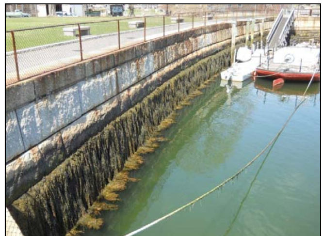
Photo 10: Quaywall at Southern End of Park
