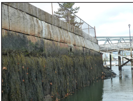
17. Quaywall Stormwater out fall.
