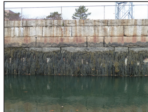
16. Quaywall Repointing existing block.
