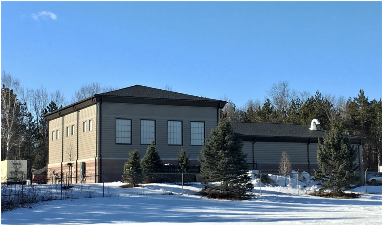
Pease Drinking Water Treatment Facility
