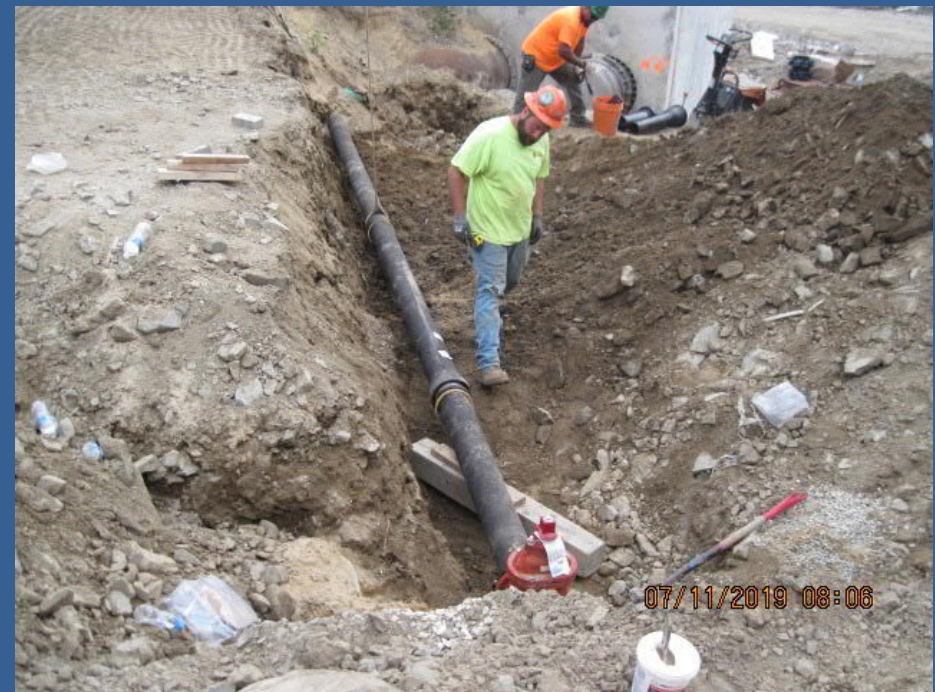
Yard Piping & Utilities
