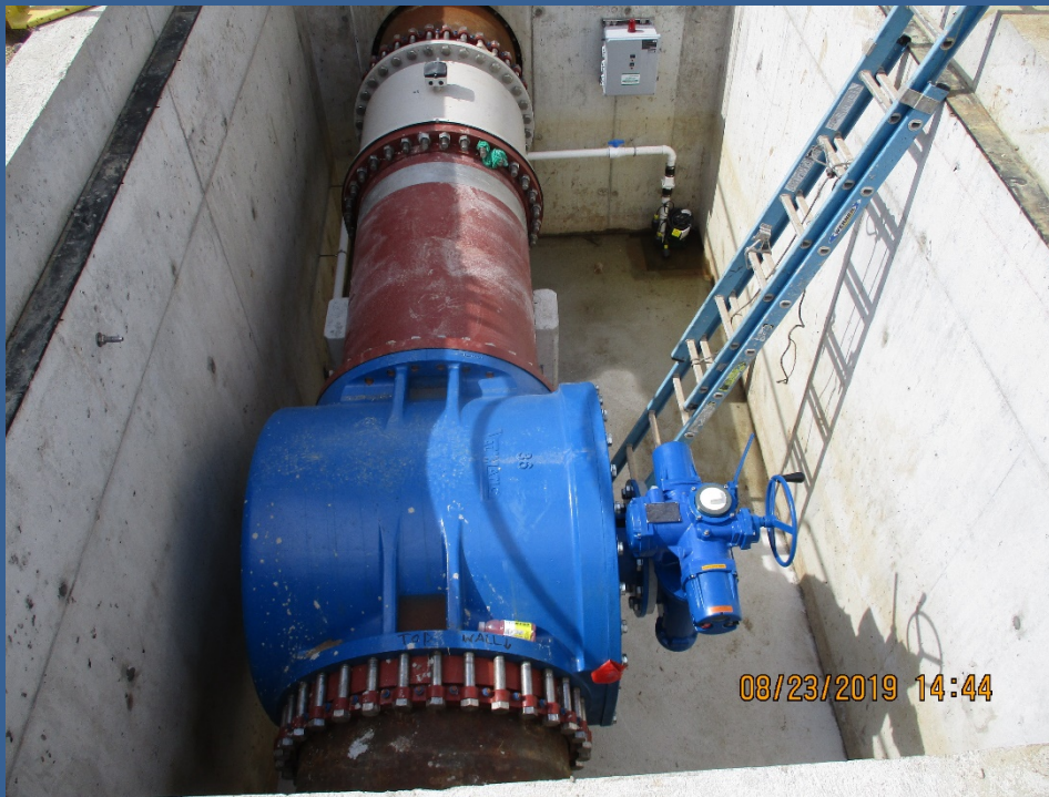
Flow Meter Vault
