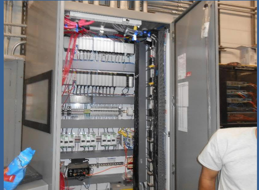
Primary Clarifier/Solids Building
