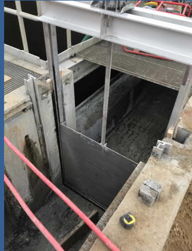
Aerated Grit Chambers
