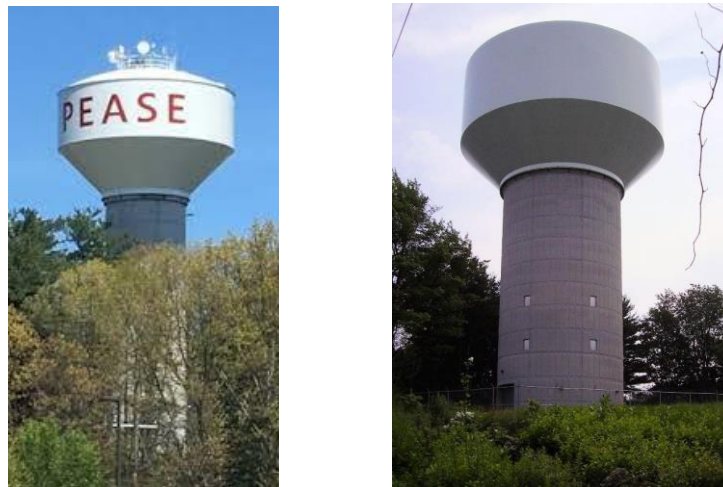
Figure C. Pease composite elevated tank (left) and Spinney Road composite elevated tank (right).
