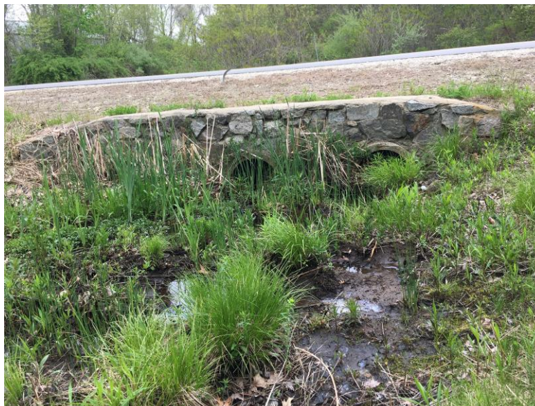
Figure 1. Three (3) 24" RCP culverts on Breakfast Hill Road.
