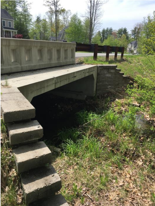
Figure 4. Example Falls Way neighborhood precast concrete box culvert.
