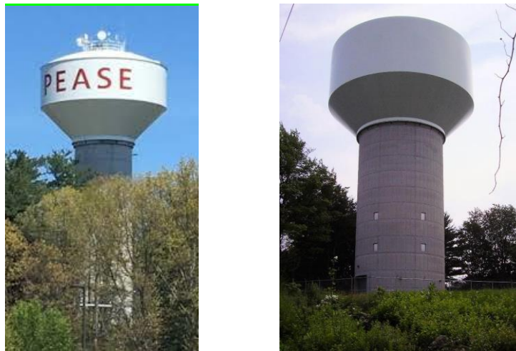
Figure 5. Pease composite elevated tank (left) and Spinney Road composite elevated tank (right).
