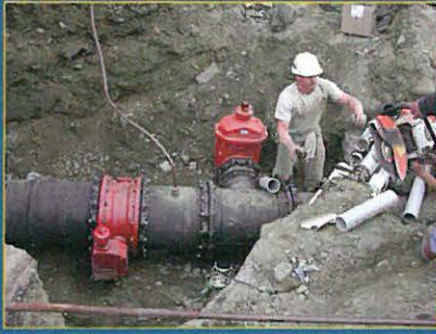
New Water Mains
