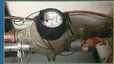
Water Meter Upgrade
