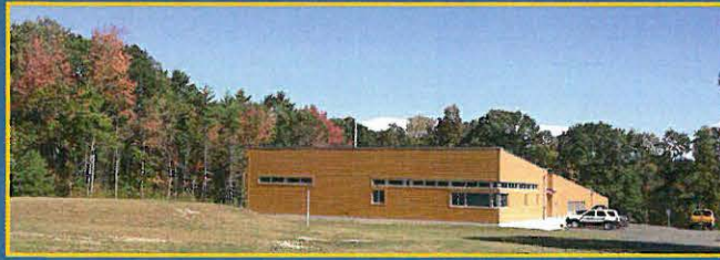
Madbury Water Treatment Facility
