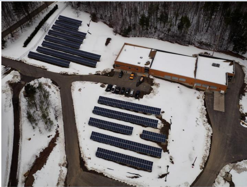
Madbury Water Treatment Plant
