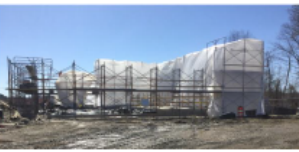
Headworks Building - Under Construction
