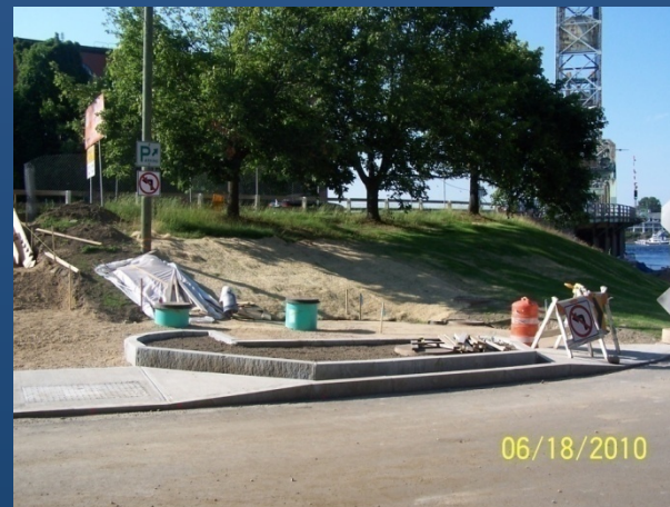
State Street Stormwater Interceptor
