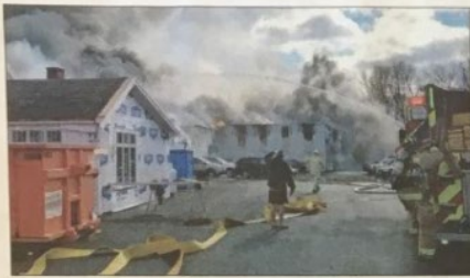
Multiple fire departments responded to a fire at Carter's European Auto Repair at 437 Portsmouth Ave. in Greenland on Saturday morning. (PHOTOS BY BUZZ DIETTERLE/SEACOASTONLINE)
