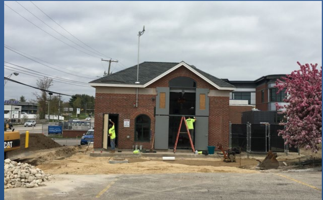
Currently under Construction
