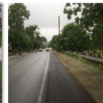
Sagamore Ave. Reconstruction with Porous Pavement
