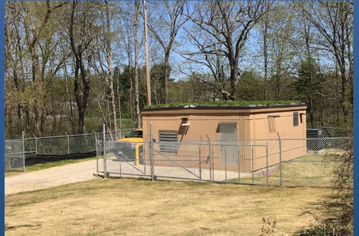
Pump Station replacement in 2017
