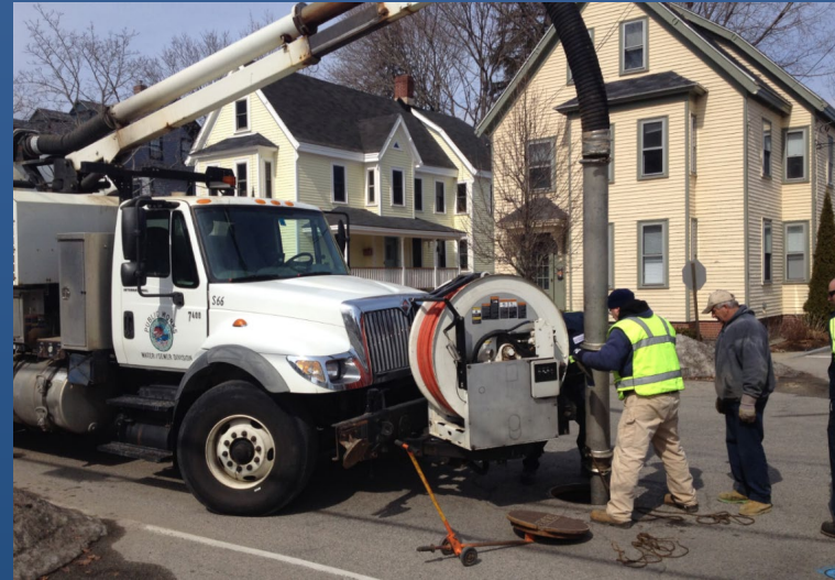
Catch Basin Cleaning - 322 Tons cleaned in 2018
