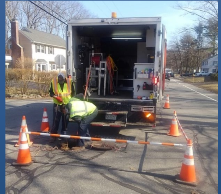
Pipe Inspections and Cleaning - 6,750 Feet Inspected and Cleaned
