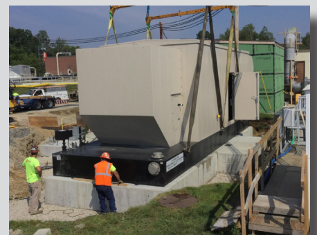
STANDBY ENGINE-GENERATOR
