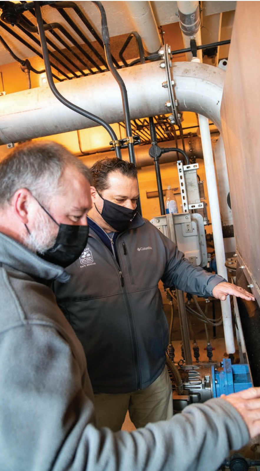
Layne DelValley (left) and Lagle check on the screenings compactor (Vulcan Industries).
