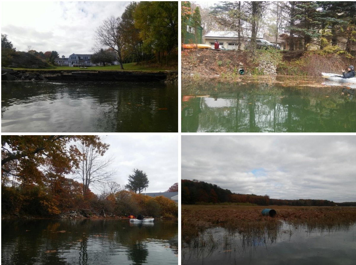
Example of collapsing retaining wall, lack of shoreline buffer, and green lawn (top left), eroding bank and unknown pipe discharge (top right), improper dumping area (bottom left), and trash/debris on marsh (bottom right). Photos taken by FBE on 11/7/2017 during the shoreline survey of Sagamore Creek.
