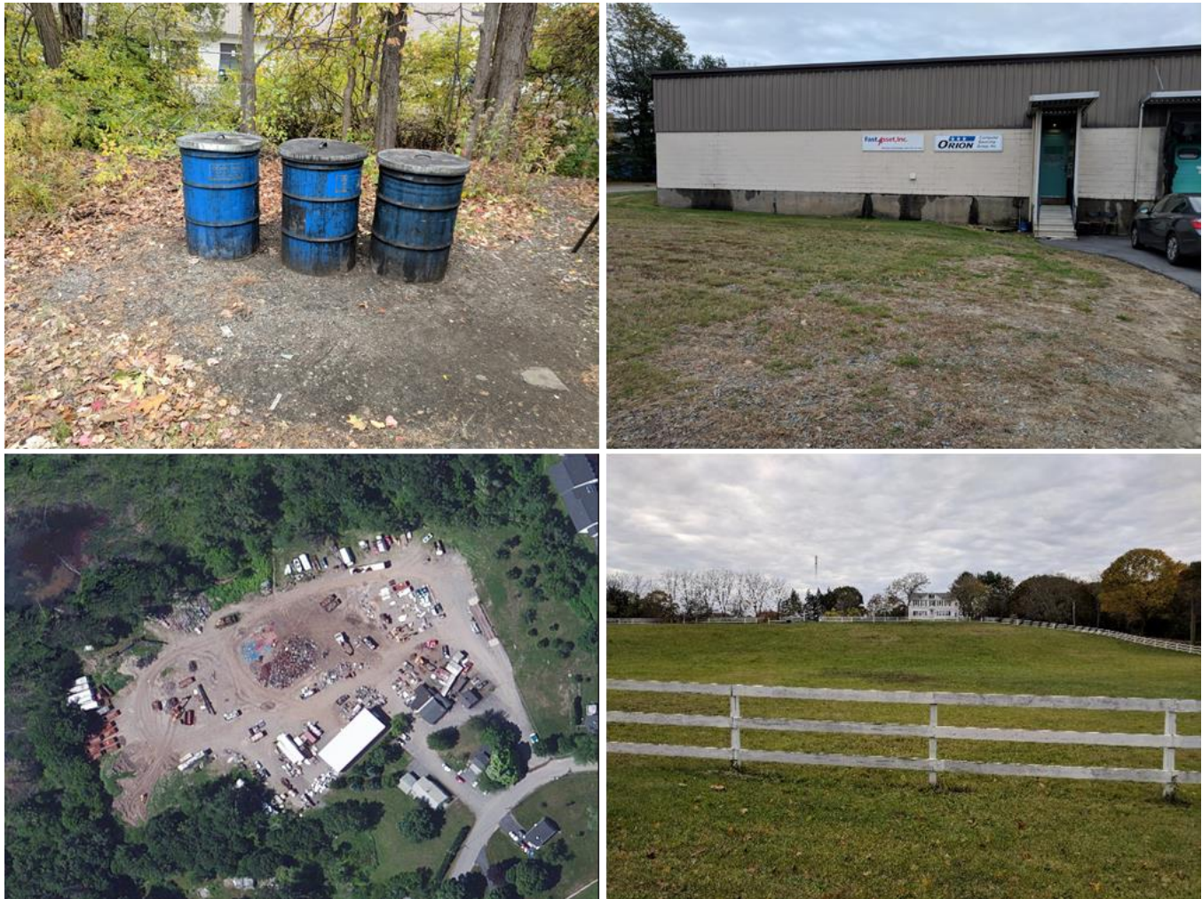
Examples of potential contamination sources identified during the 2017 watershed survey: unmarked drums outside restaurant on pervious surface (top left), seepage from unknown source identified along building foundation (top right), former scrap metal yard close to water resources (bottom left), and a horse farm on Peverly Hill Road (bottom right).
