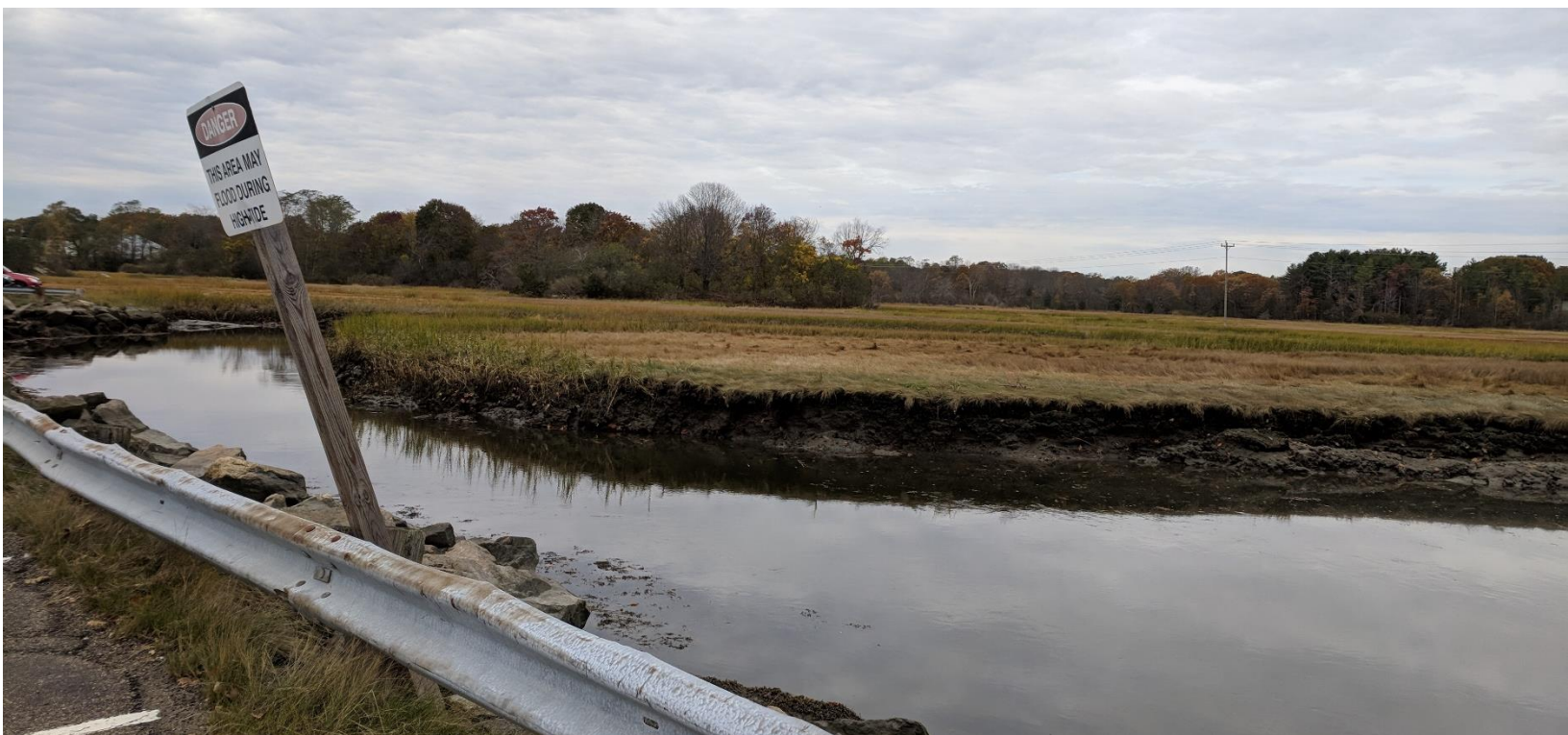
Parking lot at the Dinnerhorn restaurant just upstream of the Route 1 bridge abuts the Creek and floods during very high tides. Photo: FBE.
