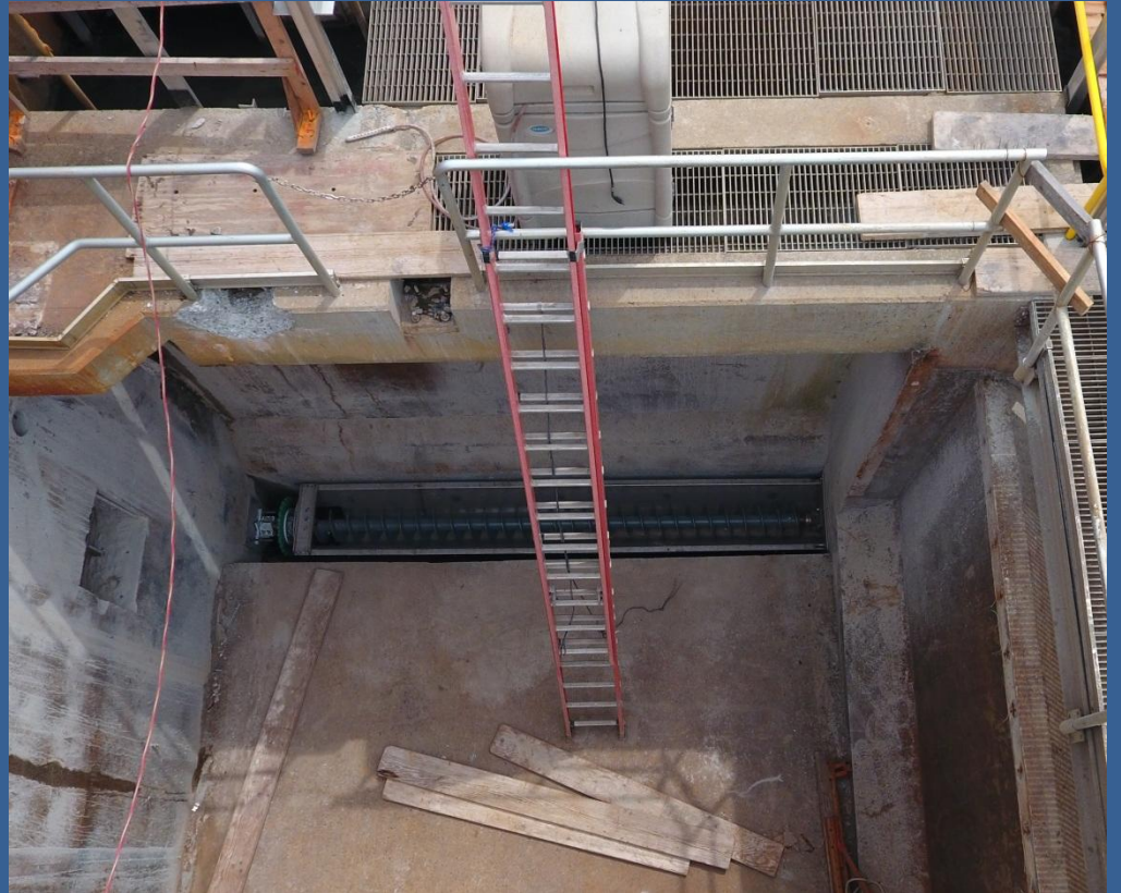
Aerated Grit Chambers
