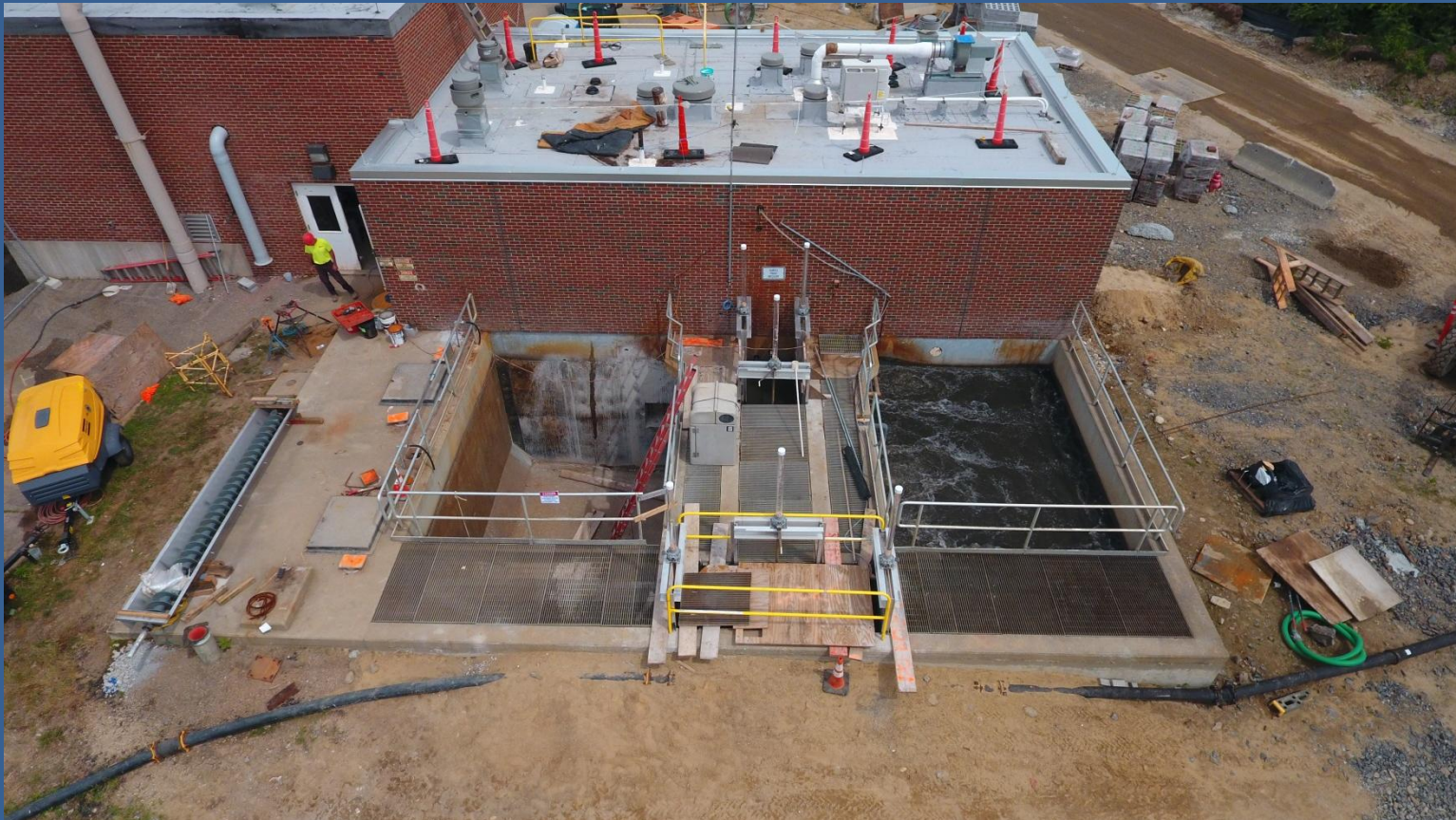
Aerated Grit Chambers
