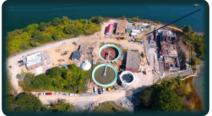
Aerial View of Peirce Island WWTF Upgrade Construction
