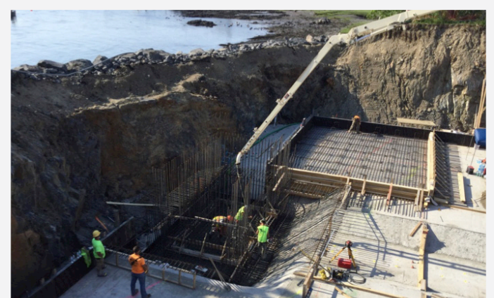
CONCRETE & REINFORCING STEEL FOR BAF BLDG APPROXIMATELY 1,200 CUBIC YARDS OF CONCRETE HAVE BEEN PLACED FOR THE BAF THROUGH JUNE 2017.
