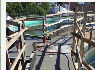
GRAVITY THICKENER NO. 2 CONCRETE PERIMETER WALKWAY
