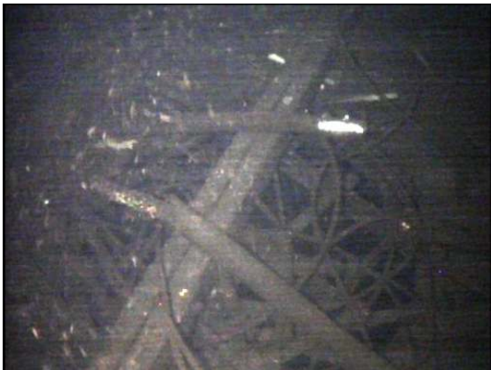
A dense network of discarded cathodic rods and cables in the base of the bowl prevented further inspection of these surfaces.
