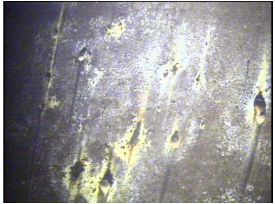
Scattered corrosion deposits along the shell and bowl surfaces where ruptured blisters are present.
