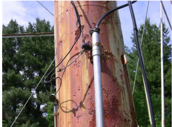
Conduits for various utility wiring along one of the support columns.
