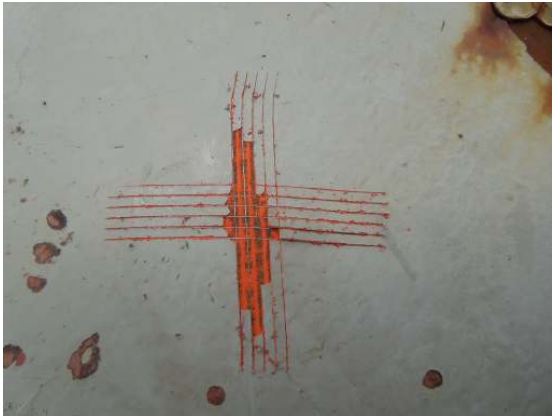
Cross hatch adhesion testing indicates poor adhesion at multiple interfaces.
