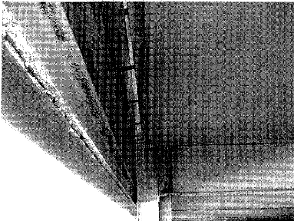
4 – Support Beam and Wall Ties (View from First Floor)
