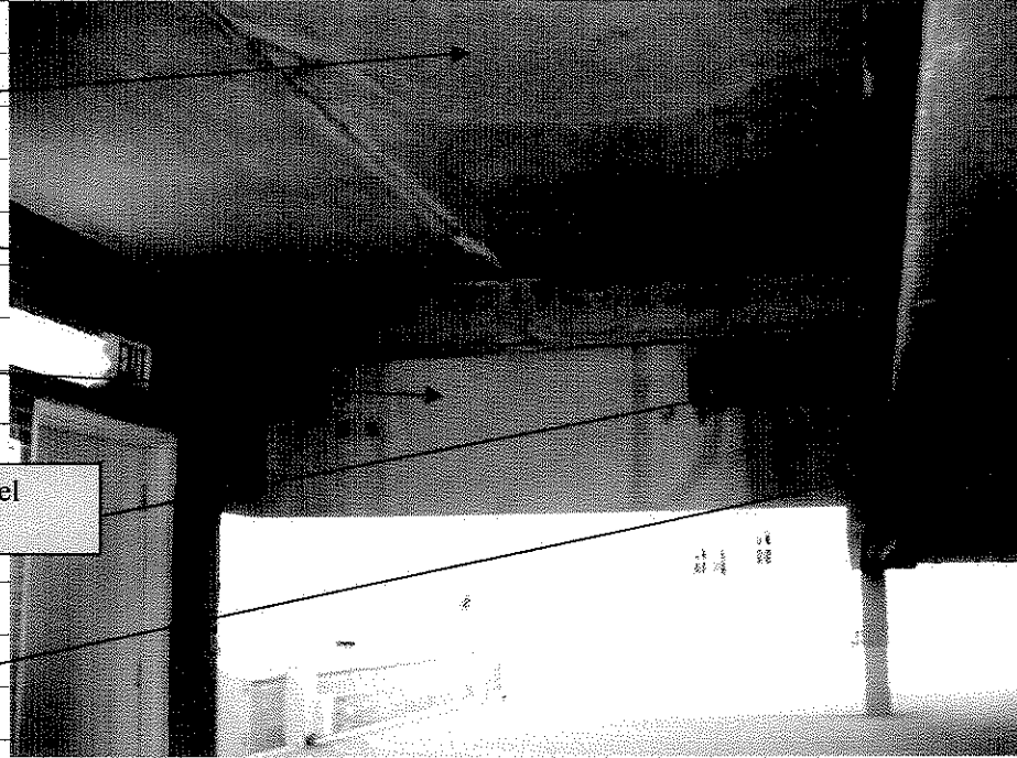
Photo#5-Elevation W12x19 at Northeast Corner-Stair Tower #1 (Grid 1.5B) and W33x152
