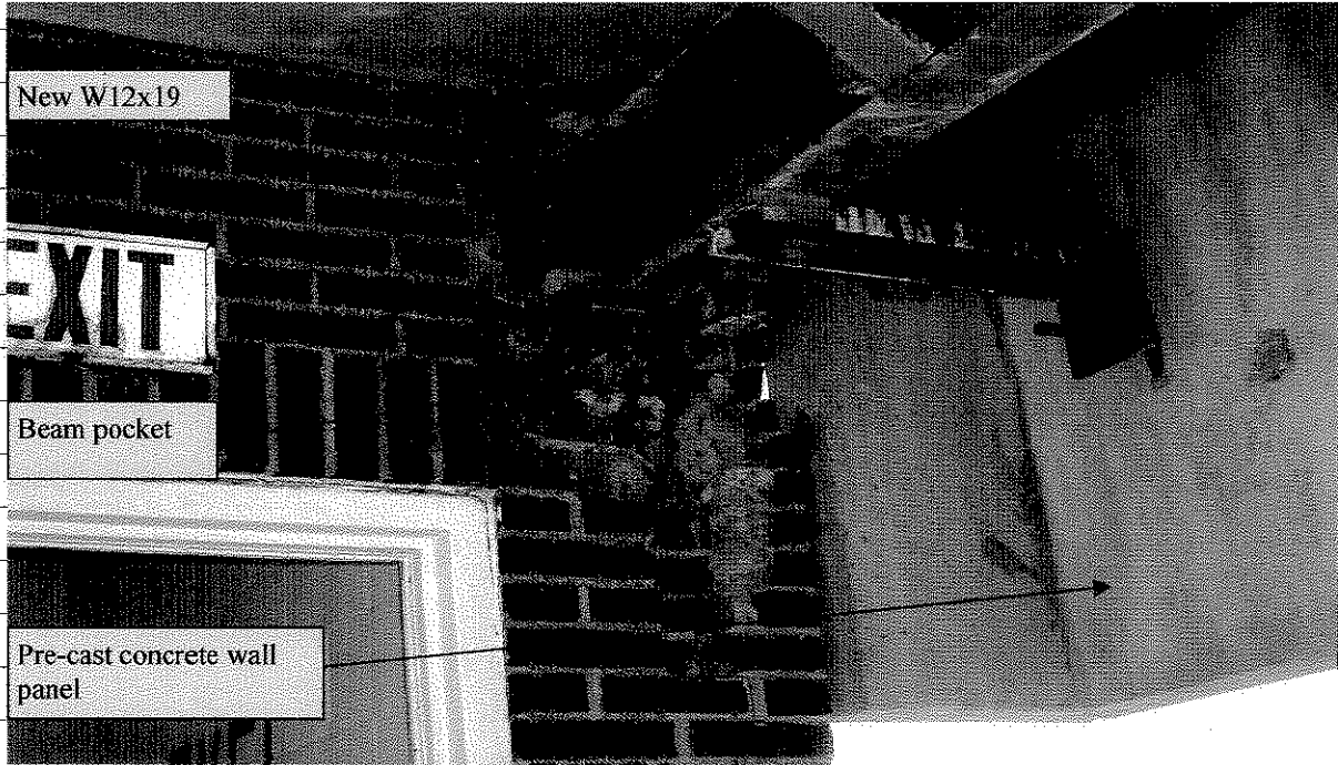
Photo#7-W12x19 at Northeast Corner-Stair Tower #1
