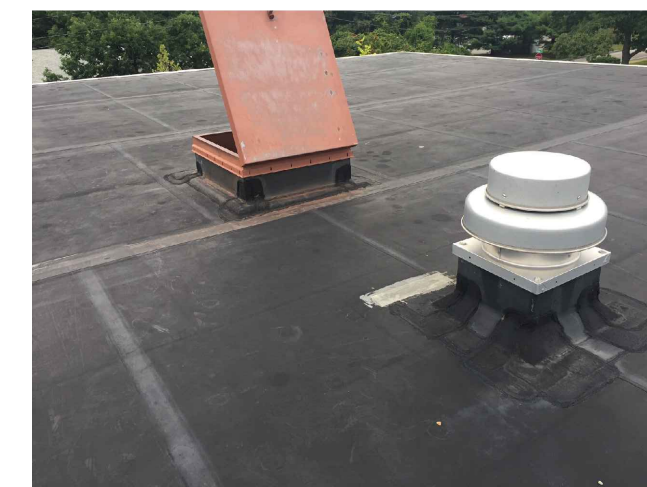
㉒ Existing Roof Hatch
