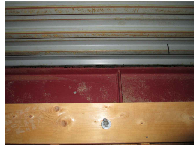
⑦ Interior Roof Soffit
