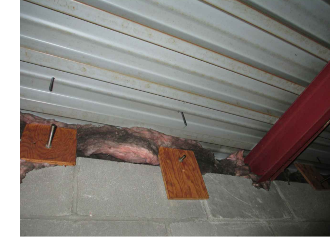
⑥ Soffit Insulation
