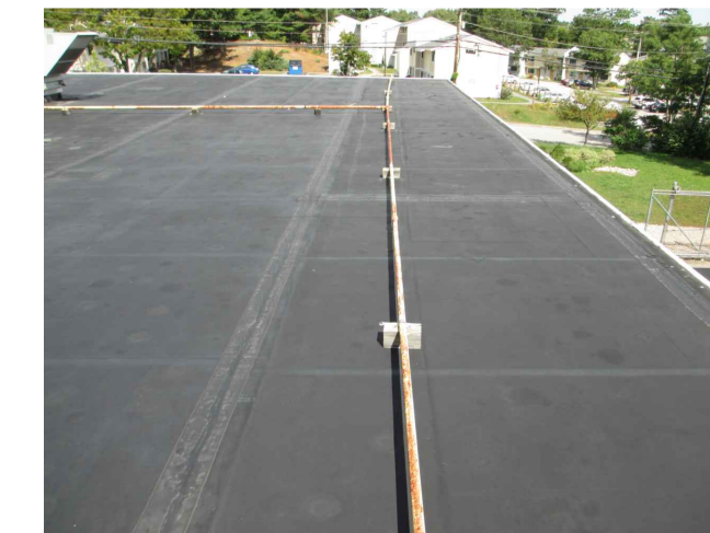
⑰ Gas Supply Piping
