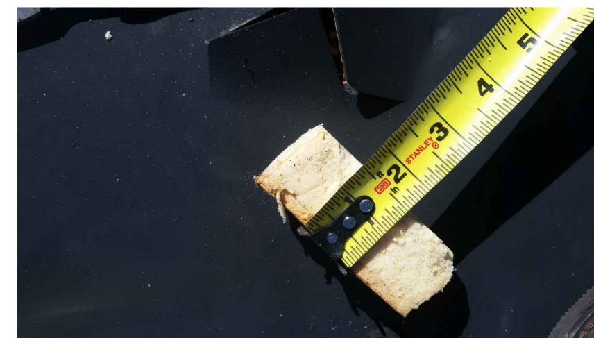
㉑ Existing Insulation
