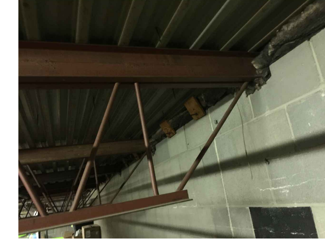
⑤ Bar Joist Detail
