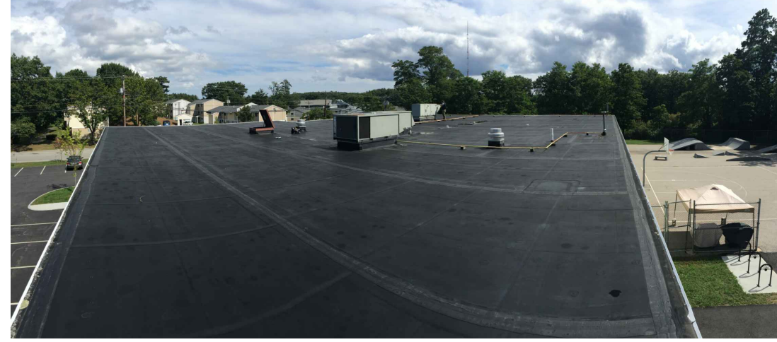
① Roof Overview (South East View)
