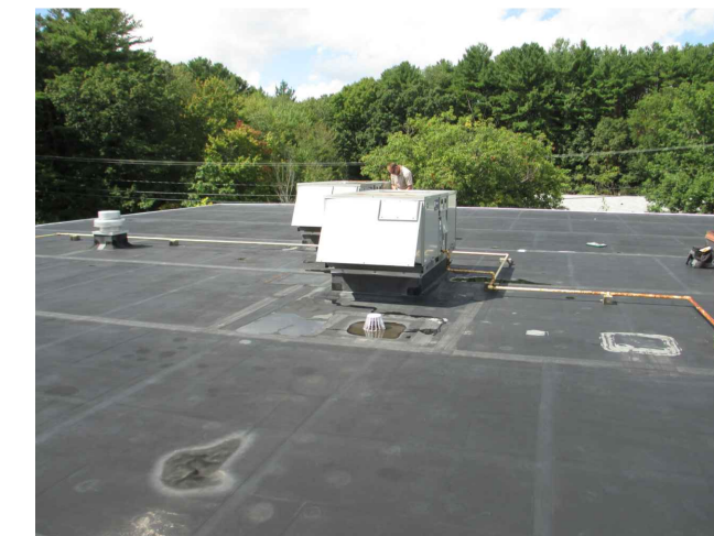
⑯ Gas Supply Piping
