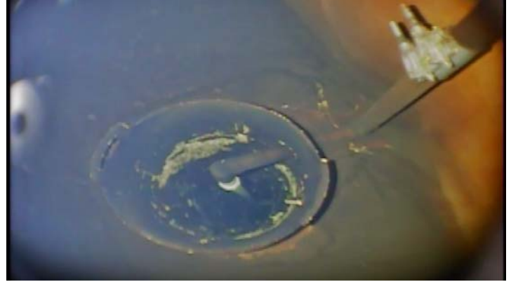
Showing feed line to bubbler system extending through site trap and down fill line
