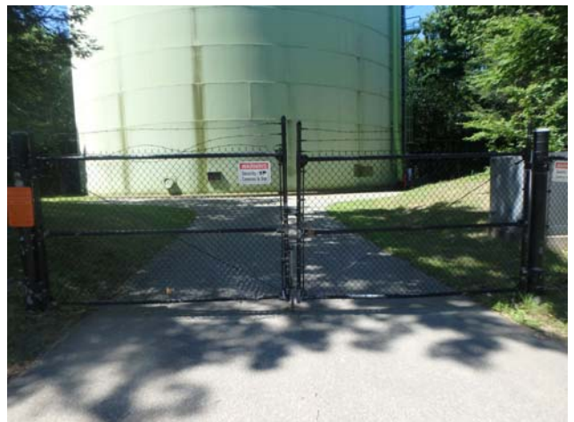
Showing the gate within the perimeter fence closed and locked post inspection
