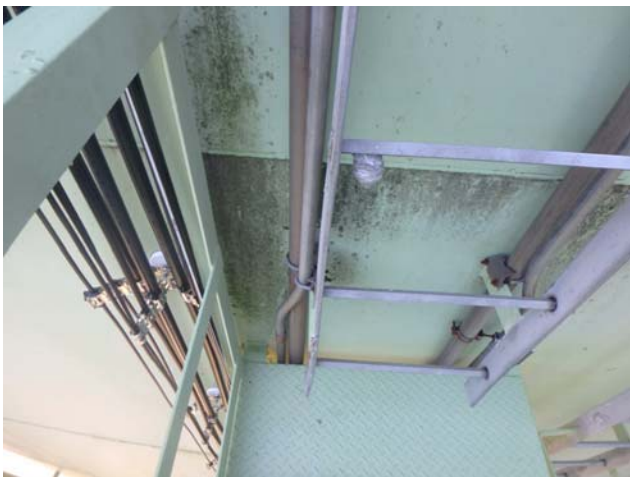
Showing presence of a small, active bee nest attached to a section of shell access ladder
