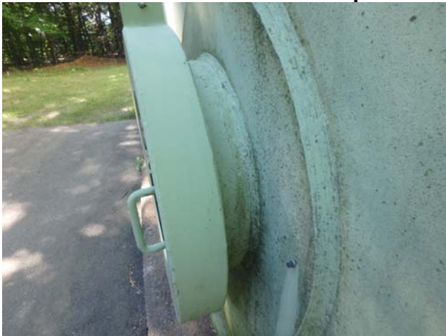
Showing typical condition of coatings along all (3) shell manholes
