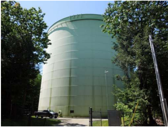
Overall view of tank exterior
