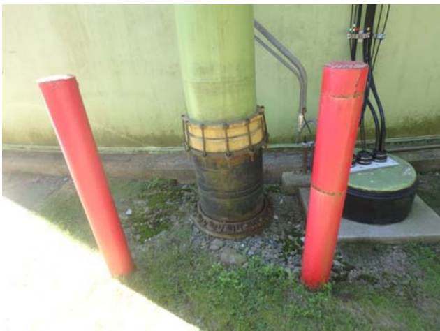
Showing overflow pipe entering directly into underground piping
