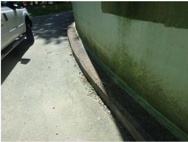
Showing foundation to be intact and in generally very good condition
