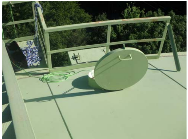
Showing primary roof hatch to be intact and structurally sound
