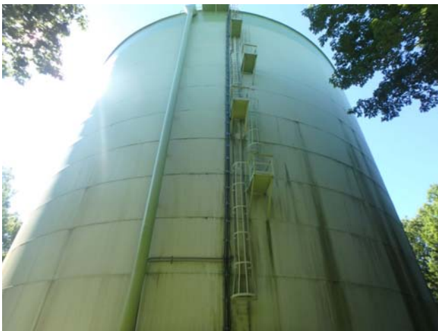
Showing overall condition of the shell coatings to be very good
