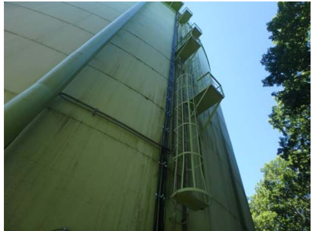
Showing entire ladder cage assembly to be intact and structurally sound
