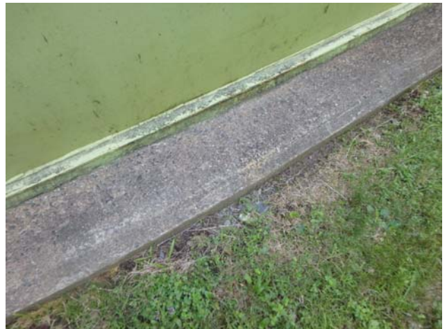
Showing concrete foundation to be in generally very good condition
