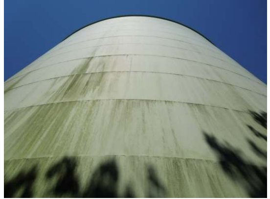
Shows little if any coating degradation occurring along the shell plates
