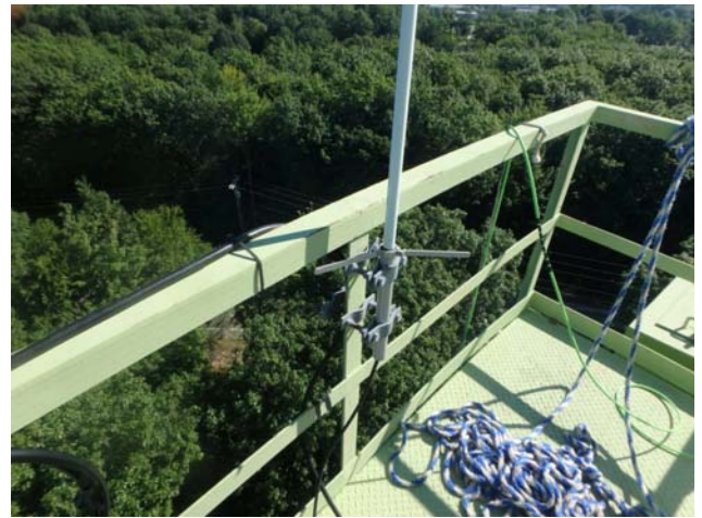
Showing platform handrail to be intact and structurally sound
