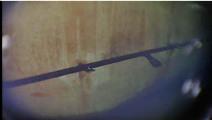
Showing the bubbler system along the interior of the bottom shell ring to be intact and in visually good condition
