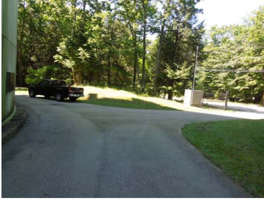
There is an asphalt drive around the perimeter of the tank
