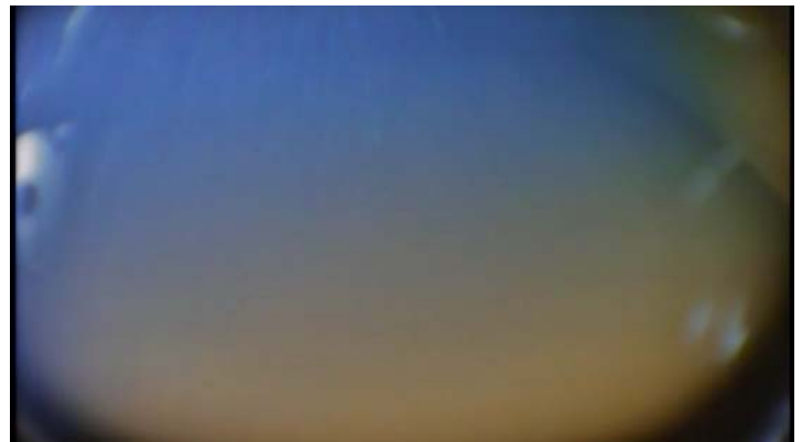
Showing floor covered with a uniform layer of sediment which impeded view of the floor surfaces
