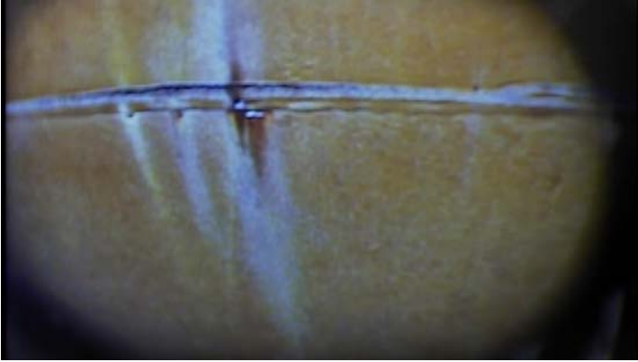
Showing isolated areas of small rust tubercle formations along interior weld seams
