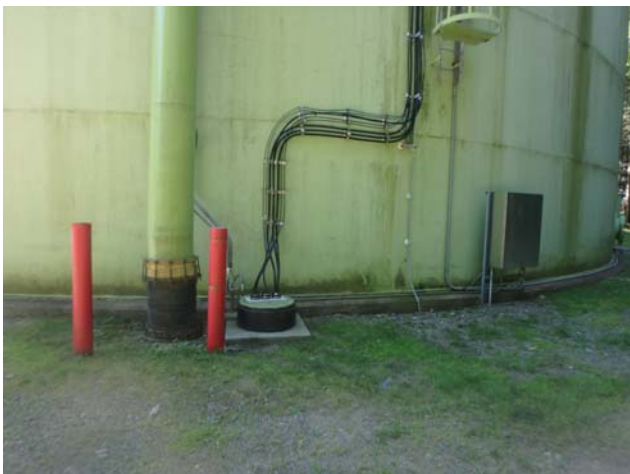
Showing shell access ladder terminating approximately 10' above grade
