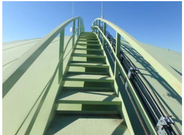
Showing roof stairway assembly to be intact and structurally sound
