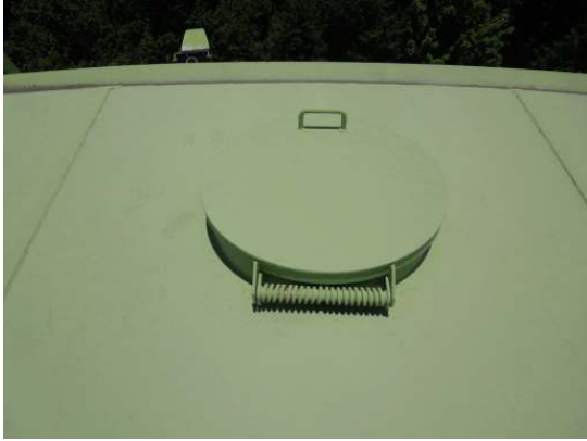
The roof hatch covers are equipped with spring hinges
