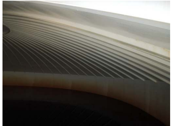
The shell surfaces above water level are stained from deposits in the water supply
