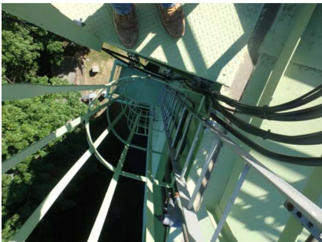
Showing stainless steel access ladder to be intact and structurally sound
