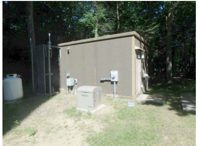
Showing the support building for the antennas atop the roof of the tank
