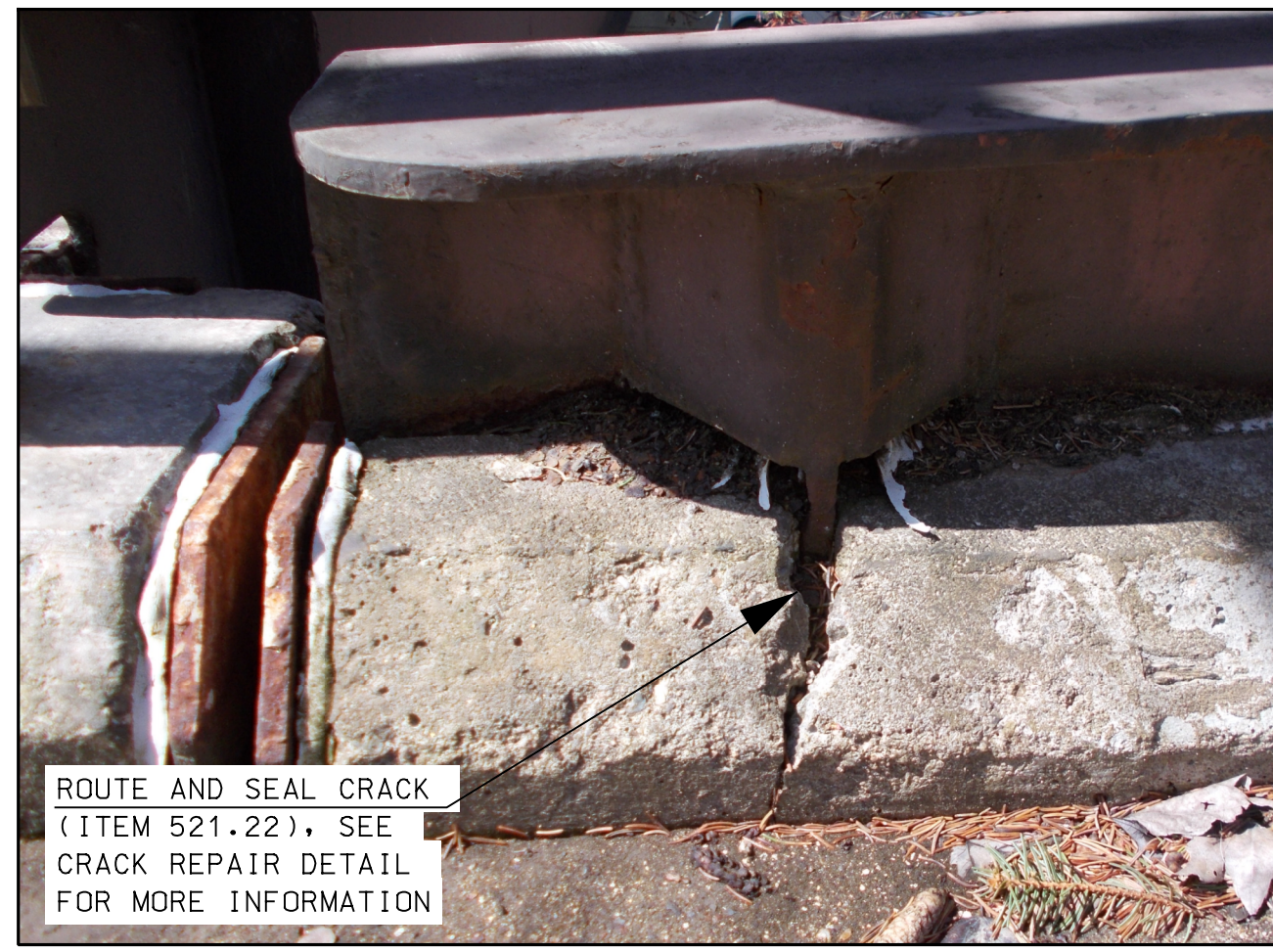
TYPICAL CRACK REPAIR NOT TO SCALE
