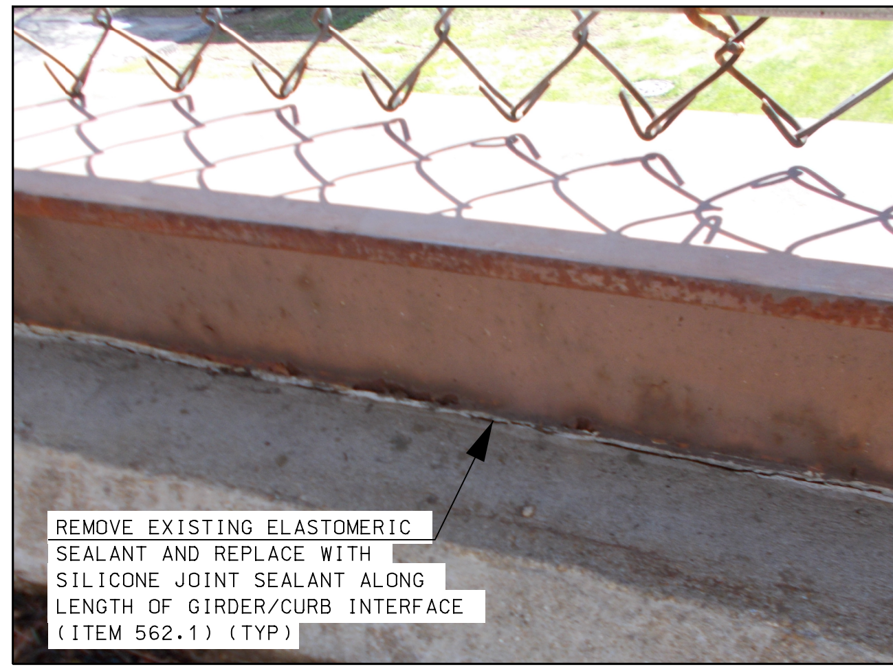
SEALANT REPLACEMENT NOT TO SCALE
