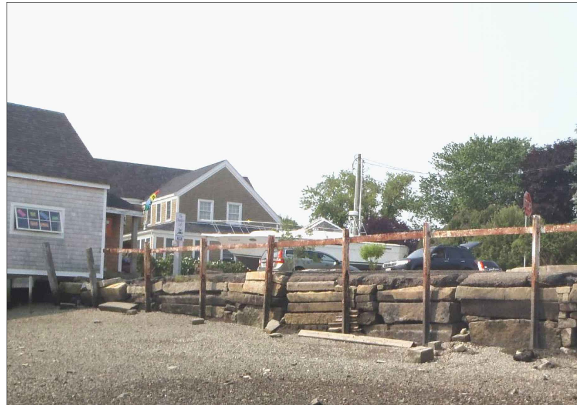
MECHANIC STREET SEAWALL (LOOKING TOWARDS SOUTH)
