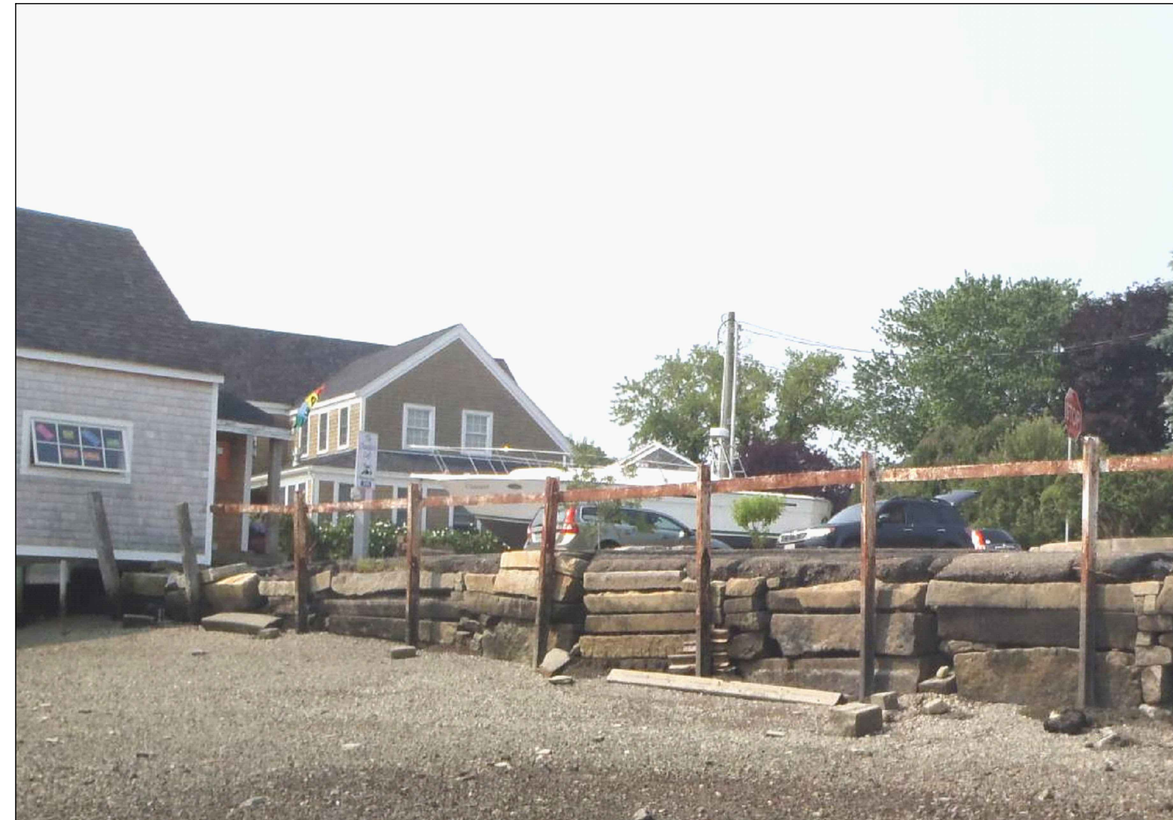
MECHANIC STREET SEAWALL (LOOKING TOWARDS SOUTH)
