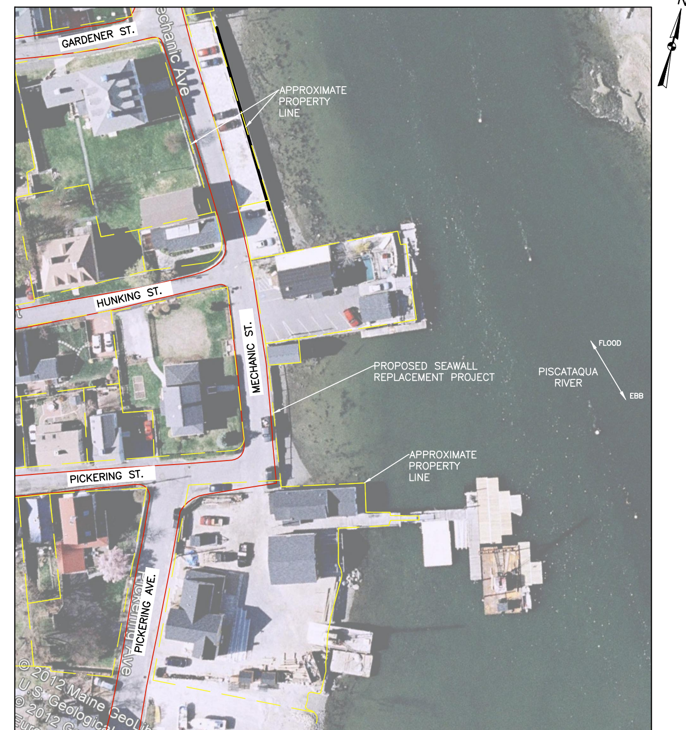
MECHANIC STREET SEAWALL AERIAL IMAGE
