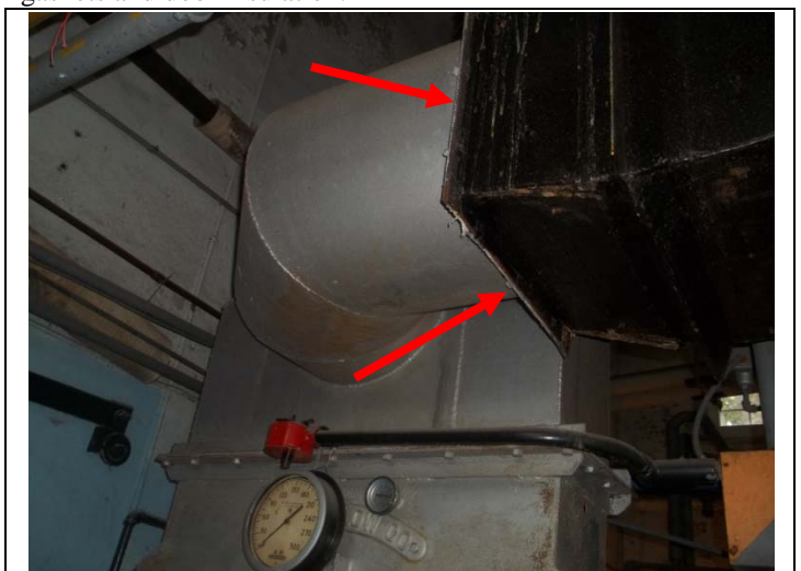
6. Square duct above boilers with ACMG gasket at flanges (arrow).
