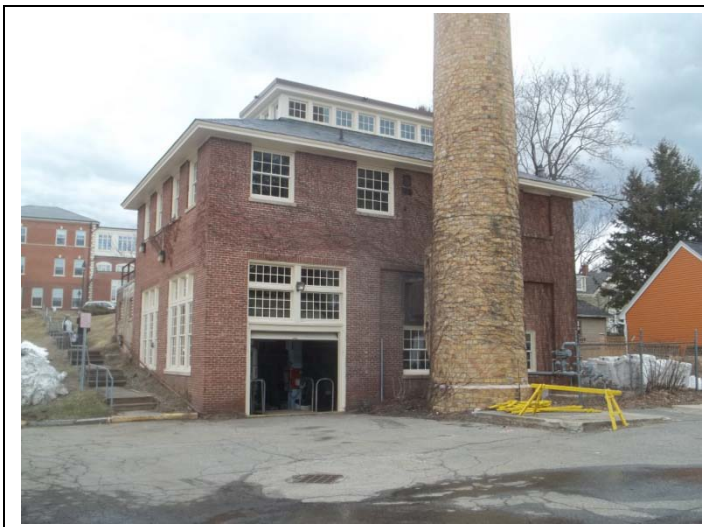
1. Exterior view of City Hall Boiler House. Overhead door access to lower level on left and exhaust stack on right.
