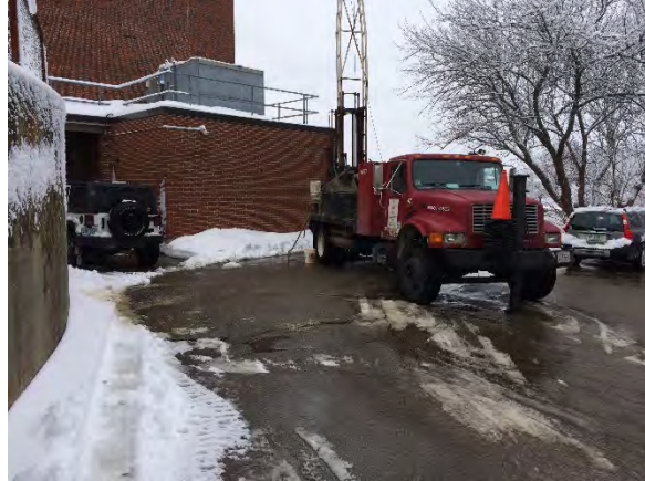
Site, To Northwest (set up at B-2)
