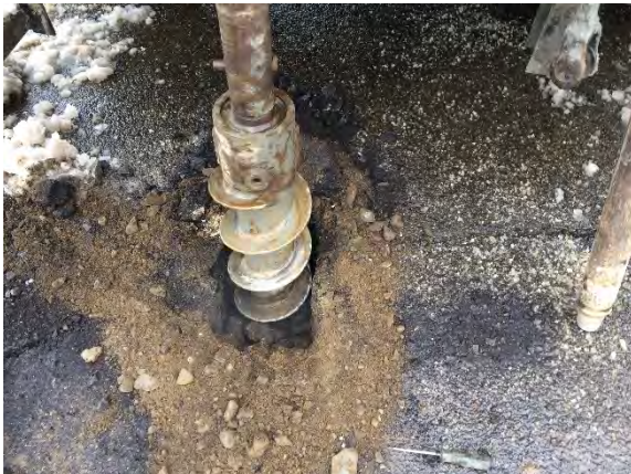
Drilling operations, Typical
