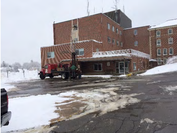
Site, To Northeast (set up at B-1)
