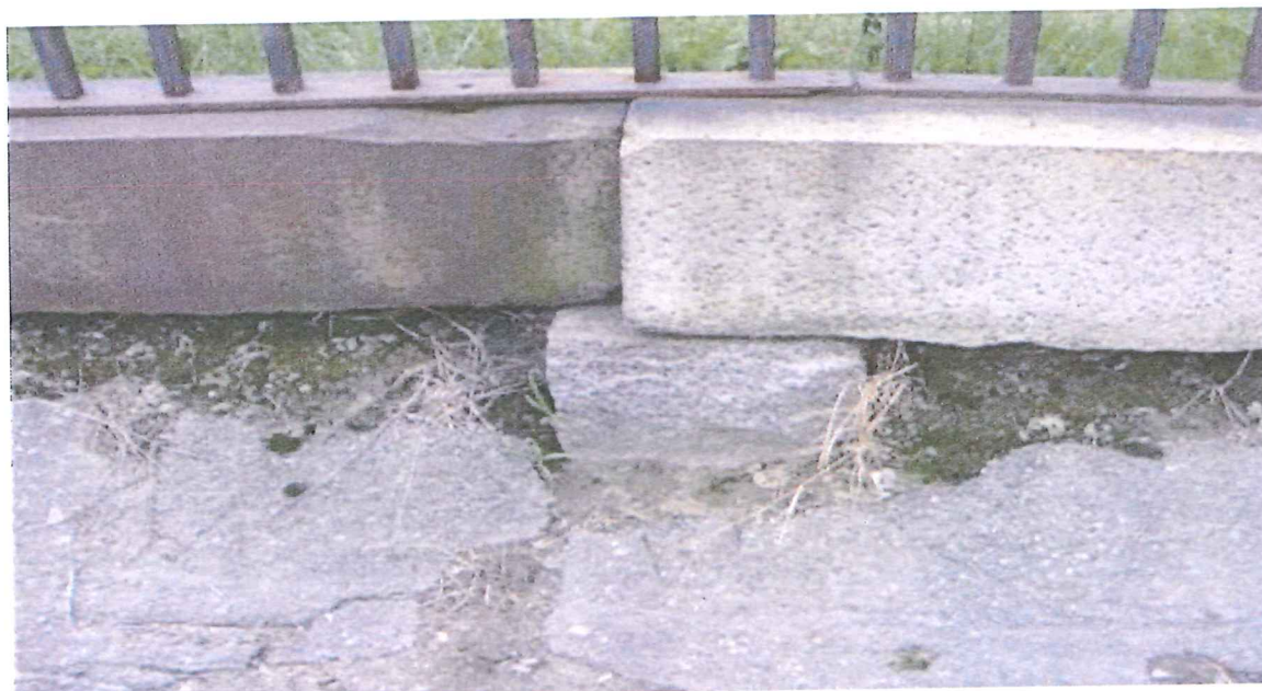
Cemetery Enclosure Fence and Stonework: Exposed wall support masonry
