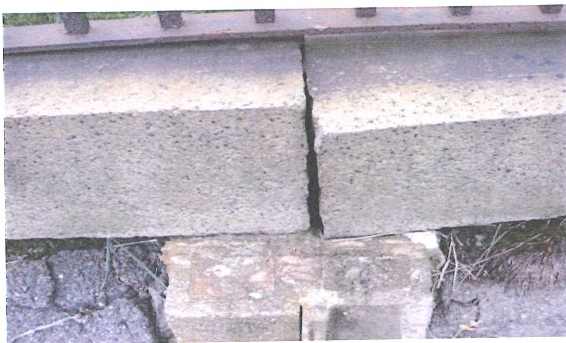
Cemetery Enclosure Fence and Stonework: Exposed wall support masonry
