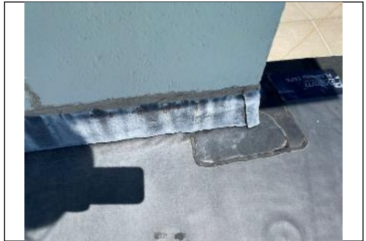
10. View of the Pump House lower roof abutment.
