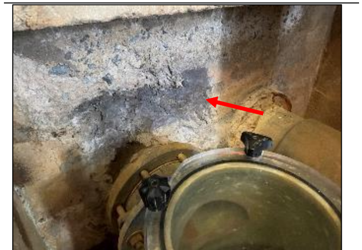
12. View of Non-ACBM dark gray patching material on wall in Pump House.
