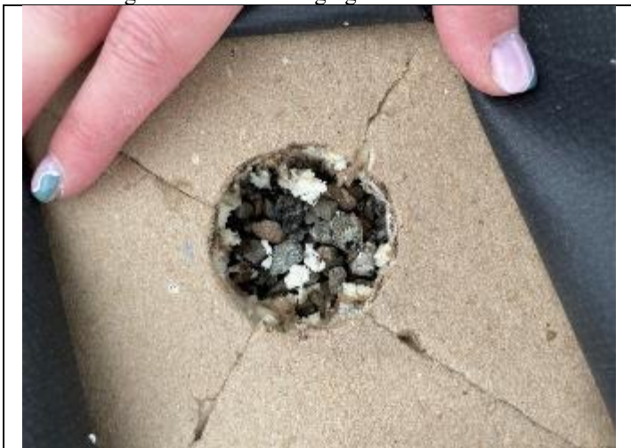
5. View of the roof core sample on the Bath House roof.
