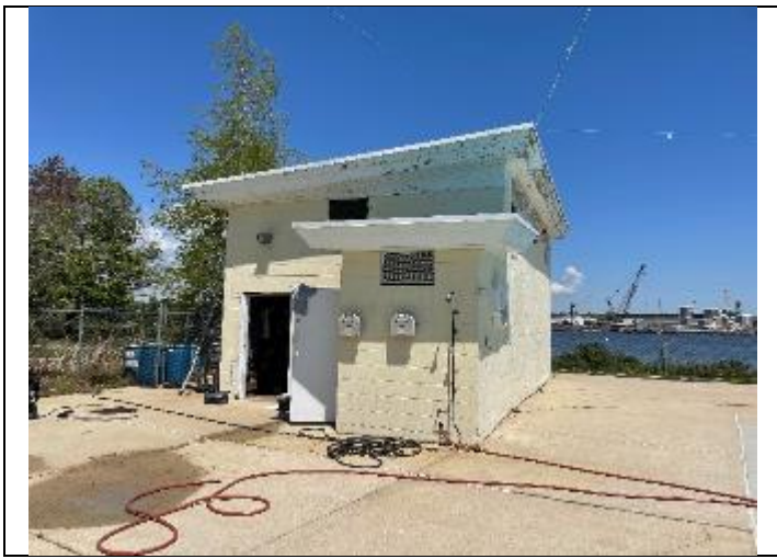
7. Exterior view of the Pierce Island Pump House.
