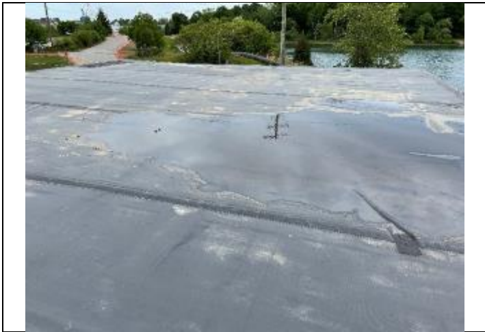
9. View of the upper roof of the Pump House.
