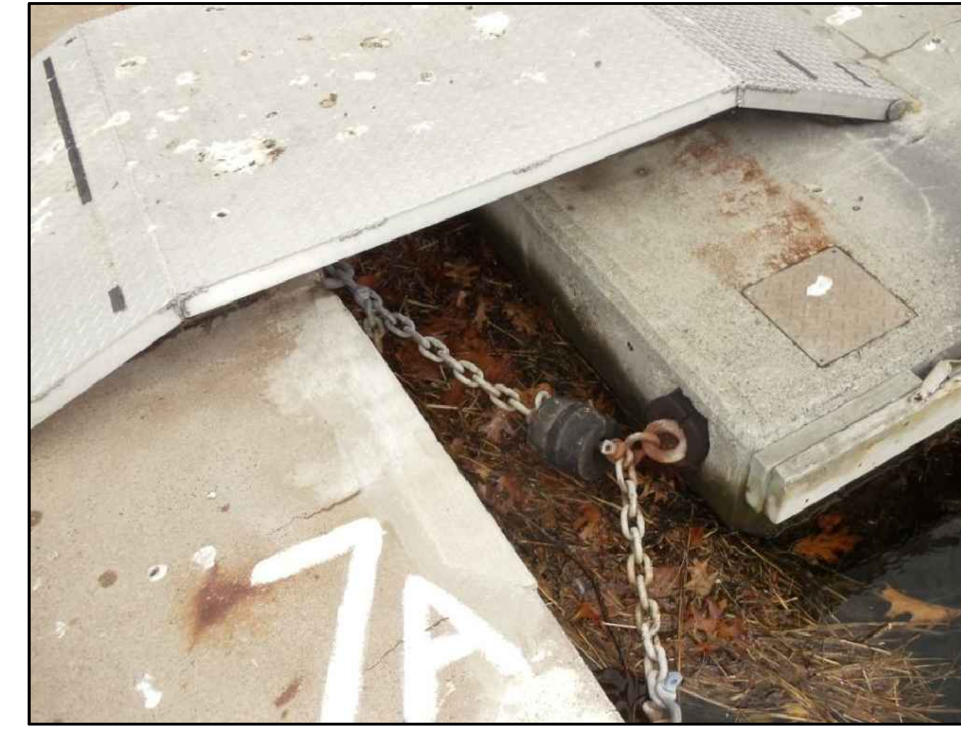
3 EXISTING FLOATING DOCK CONNECTION
