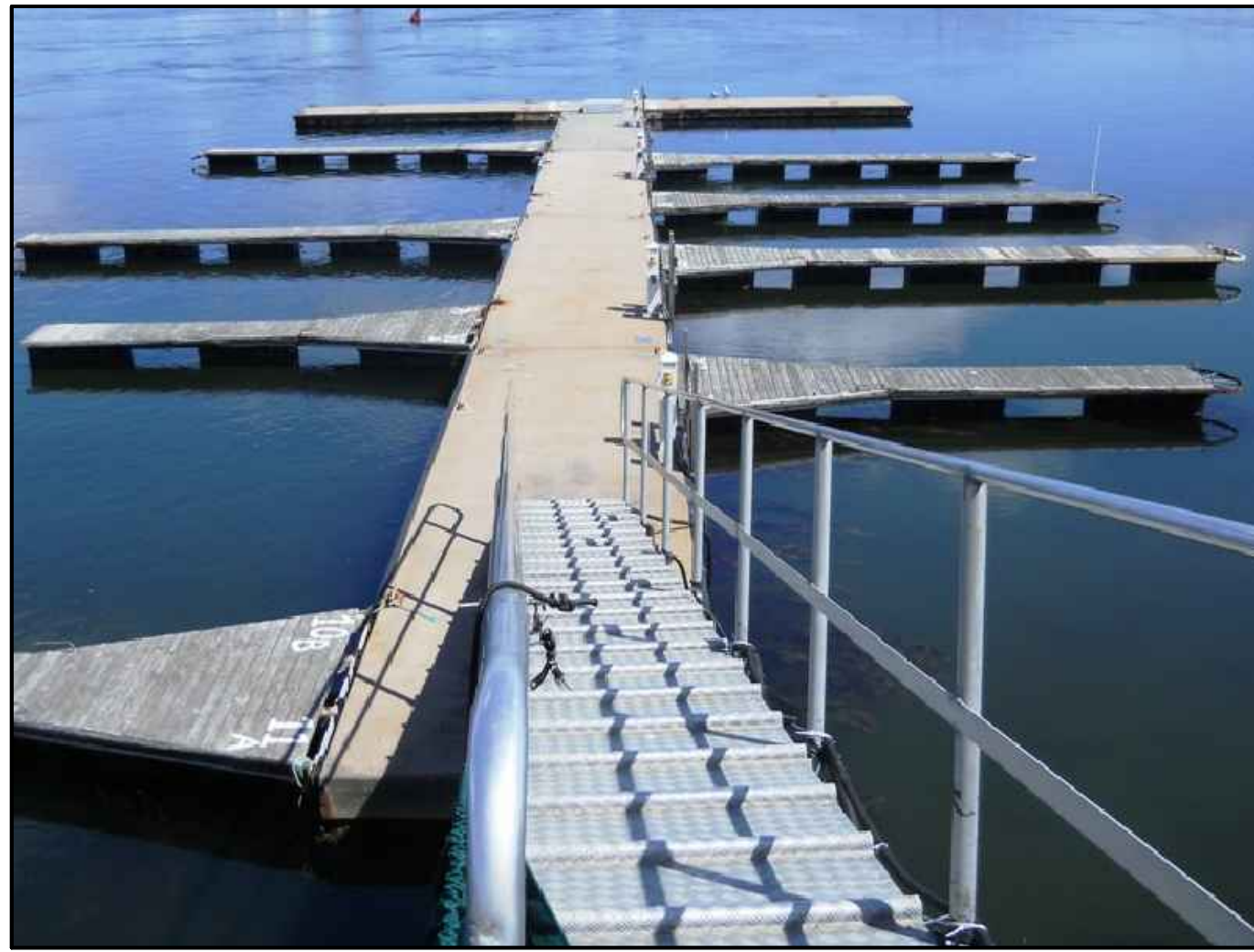
1 EXISTING FLOATING DOCK OVERALL
