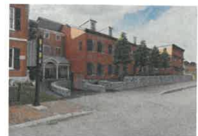
93 Pleasant Street – Deep energy Retrofit & Addition, Offices – reduce energy usage by 60% beyond standard baseline.
