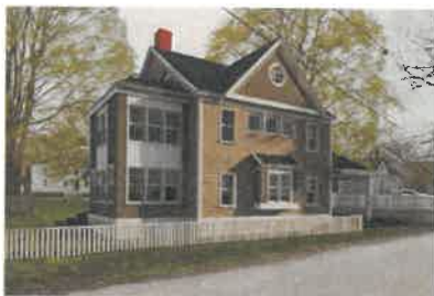
Fishmonger Cottages – Net Zero subdivision with new construction single family homes.
